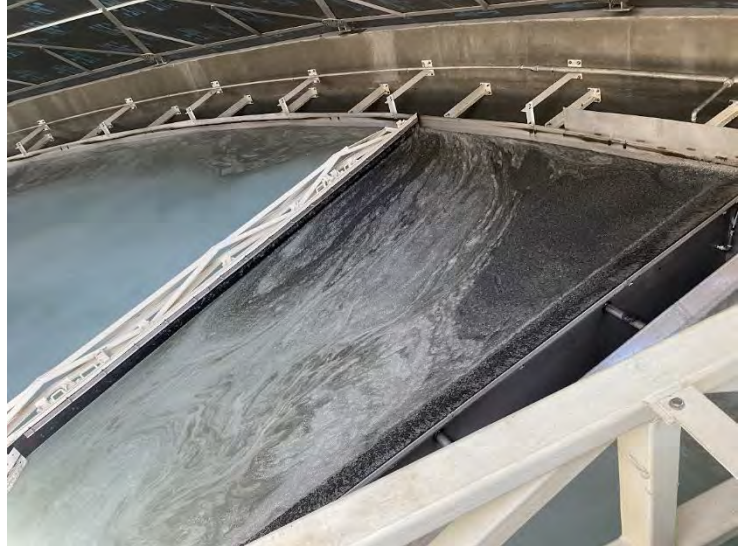
71. DAF No. 1 Tank: SAT for In-Service Mode / Full Flow to Filters (2022-09-08)
