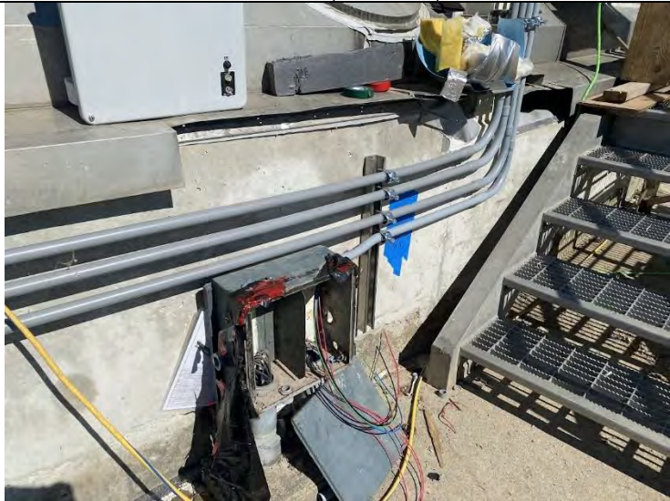
64. DAF No. 1 Tank to Blowdown Chamber Conduit (2022-09-08)
