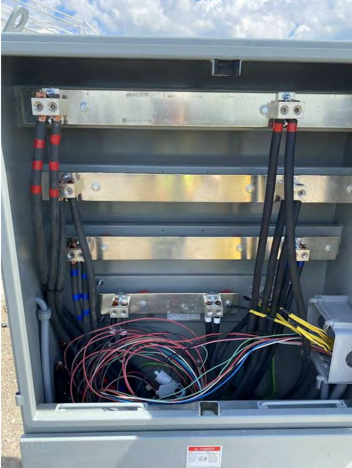
33. Generator Quick Connect Panel (2022-09-07)
