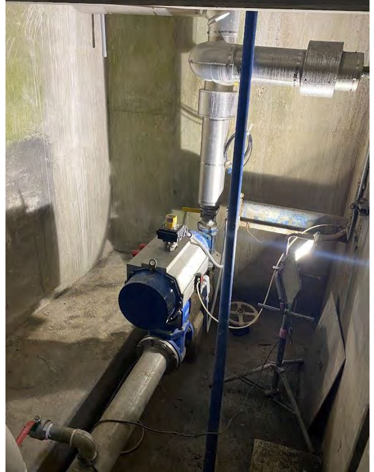
6. DAF No. 1 Blowdown Chamber: Sludge Blowdown (2022-09-06)
