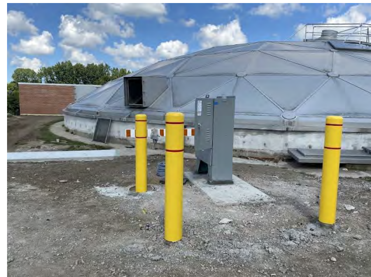
31. Generator Quick Connect Panel and Bollards (2022-09-07)
