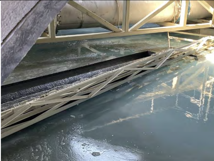
74. DAF No. 1 Tank: SAT for In-Service Mode / Full Flow to Filters (2022-09-08)
