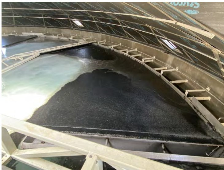
82. DAF No. 1 Tank: Significant Scum/PAC Build Up In-Service Mode (2022-09-09)
