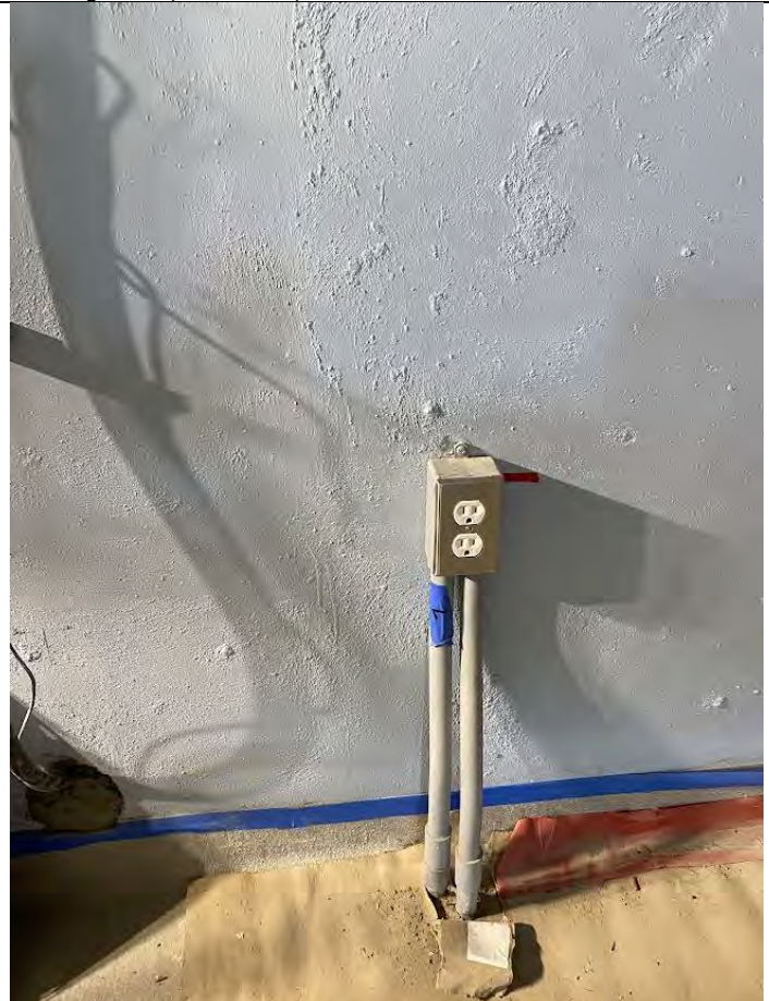
16. Auxiliary Equipment Building: Duplex Receptacle (2022-09-06)
