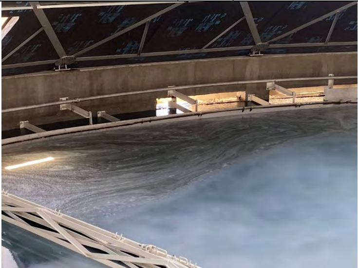
65. DAF No. 1 Tank: Switching from Partial Flow to Full Flow to Filters (2022-09-08)
