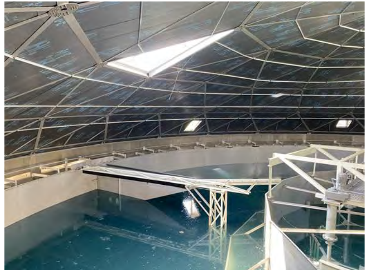
40. DAF No. 1 Tank Drained Slightly for Skimmer & Trough Modifications (2022-09-07)
