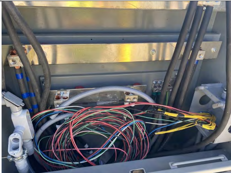
62. Generator Quick Connect Panel (2022-09-08)
