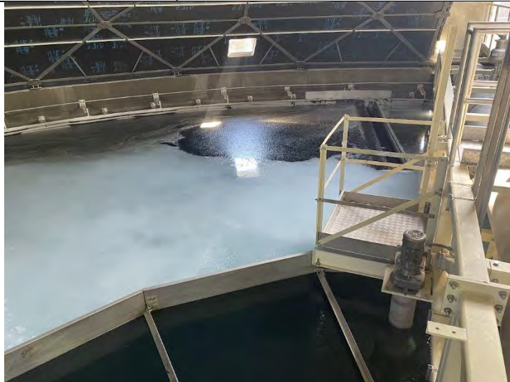
84. DAF No. 1 Tank: Significant Scum/PAC Build Up In-Service Mode (2022-09-09)
