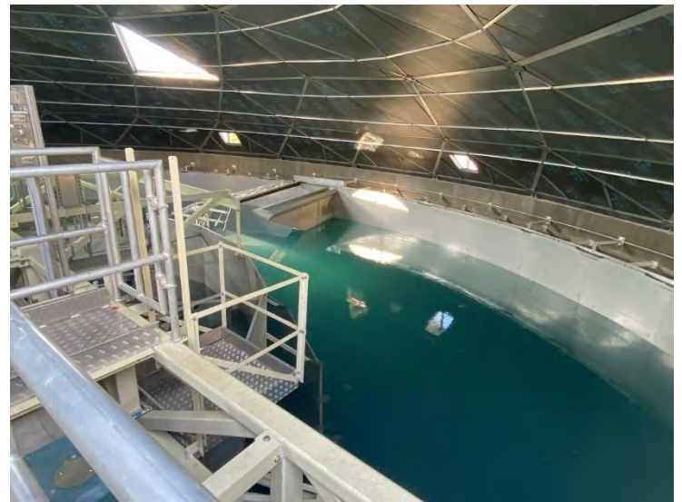
24. DAF No. 1 Tank: Slightly Drained to below Effluent Troughs (2022-09-06)
