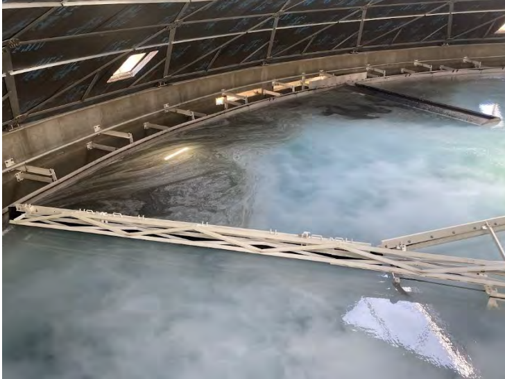
70. DAF No. 1 Tank Effluent Troughs: SAT for In-Service Mode / Full Flow to Filters (2022-09-08)
