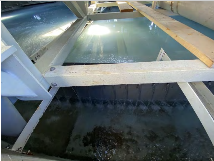
68. DAF No. 1 Tank Effluent Troughs: SAT for In-Service Mode / Full Flow to Filters (2022-09-08)
