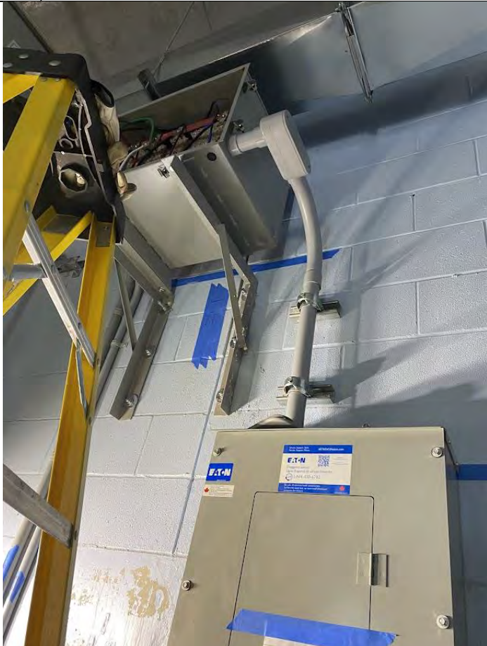
15. Auxiliary Equipment Building: Transformer and Lighting Panel (2022-09-06)
