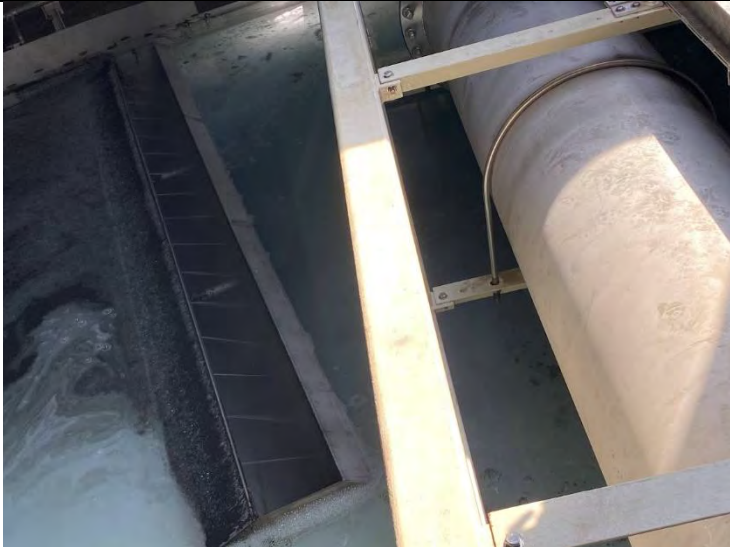
76. DAF No. 1 Scum Troughs Rinse: SAT for In-Service Mode / Full Flow to Filters (2022-09-08)
