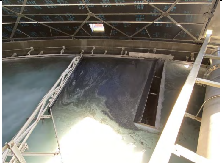
75. DAF No. 1 Tank: SAT for In-Service Mode / Full Flow to Filters (2022-09-08)
