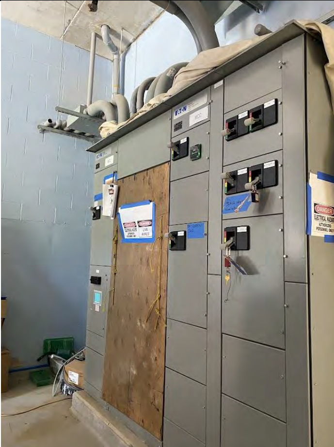
17. Auxilairy Equipment Building: MCC Pending Modifications for ATS (2022-09-06)
