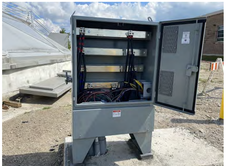
32. Generator Quick Connect Panel (2022-09-07)
