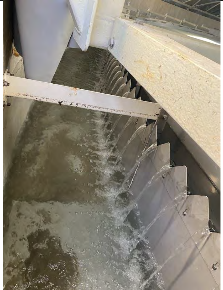
67. DAF No. 1 Tank Effluent Troughs: SAT for In-Service Mode / Full Flow to Filters (2022-09-08)
