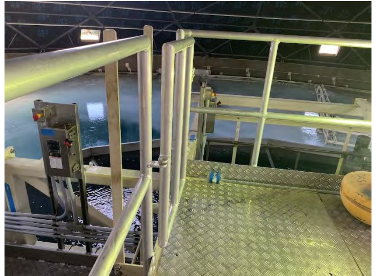
50. DAF No. 1: Lower Platform Gates Corrected (to align to close properly) (2022-09-08)
