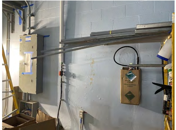
14. Auxiliary Equipment Building: Lighting Panel, Water Service Line and Fire Extinguisher (2022-09-06)
