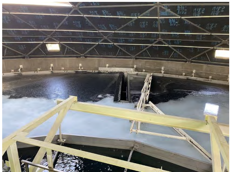
83. DAF No. 1 Tank: Significant Scum/PAC Build Up In-Service Mode (2022-09-09)
