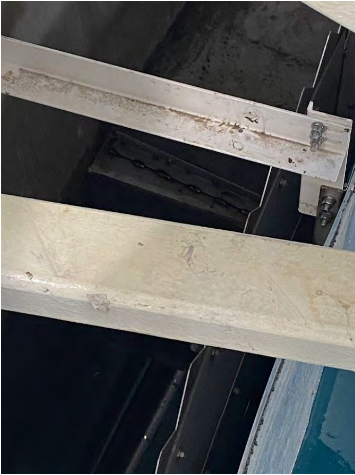
43. DAF No. 1 Tank: Effluent Trough Modifications (2022-09-07)
