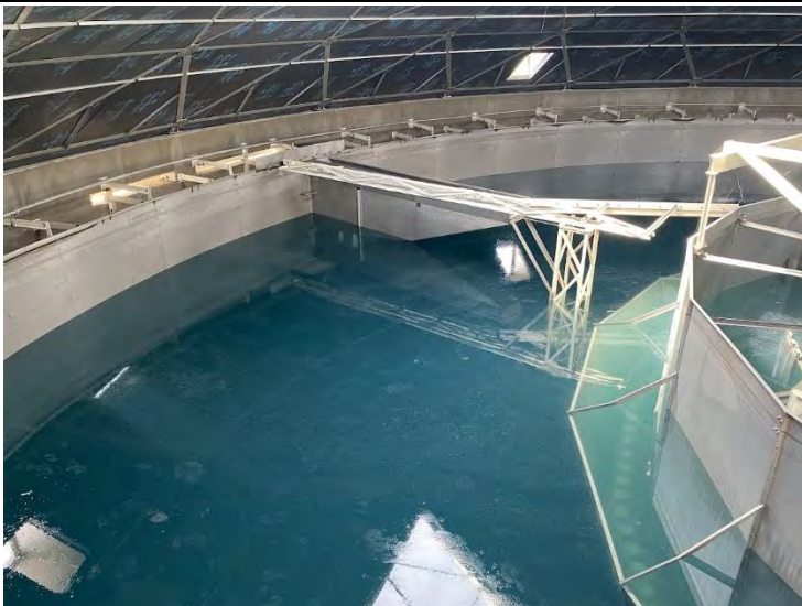
19. DAF No. 1 Tank: Slightly Drained to below Effluent Troughs (2022-09-06)
