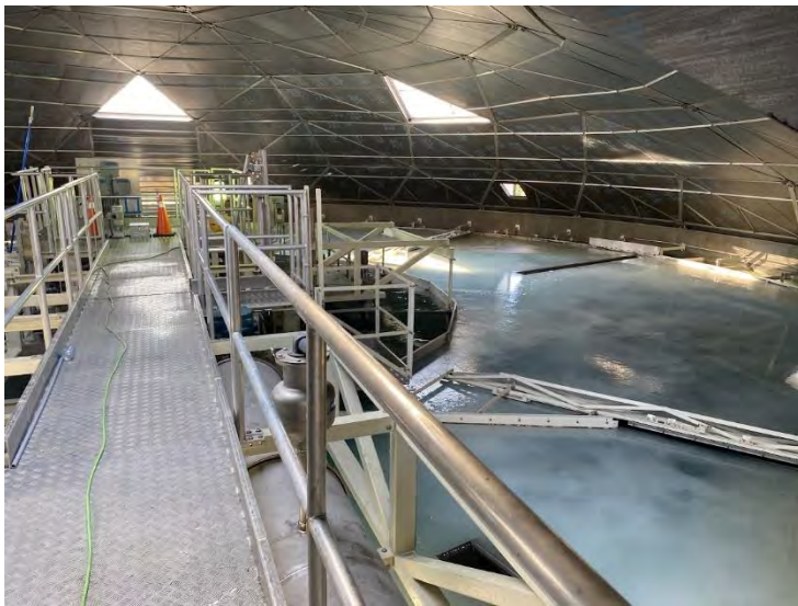
45. DAF No. 1 Tank: Partial Flow / Flow to Overflow Chamber (2022-09-07)
