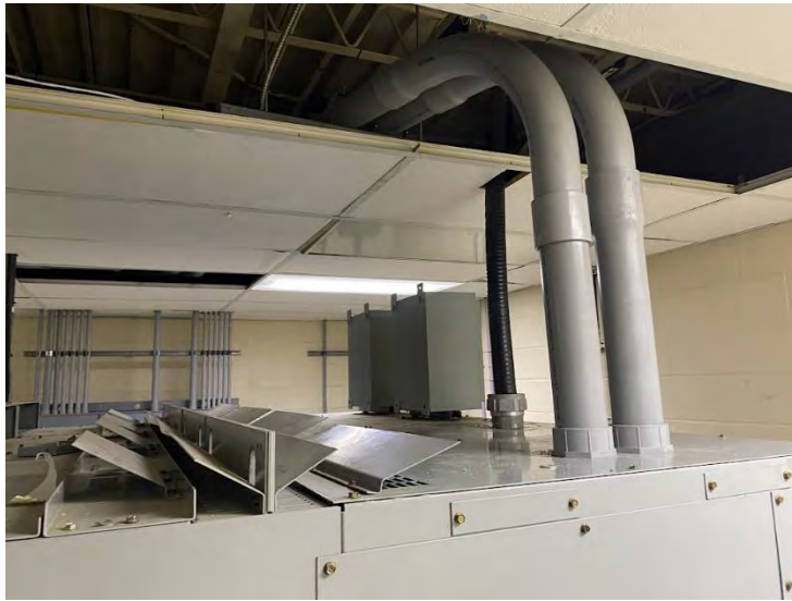
21. Ruthven WTP – Switchgear with new Conduit for DAF (2022-07-04)
