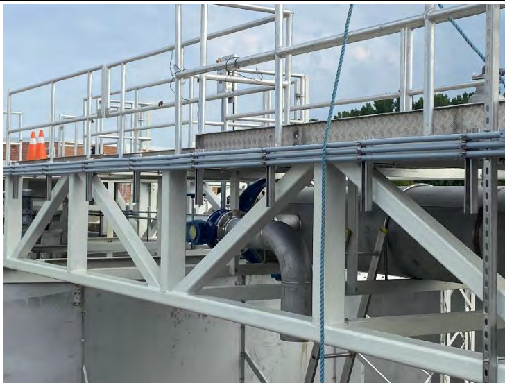
55. DAF No. 1 Tank: Influent Piping Bypass Line (2022-07-08)
