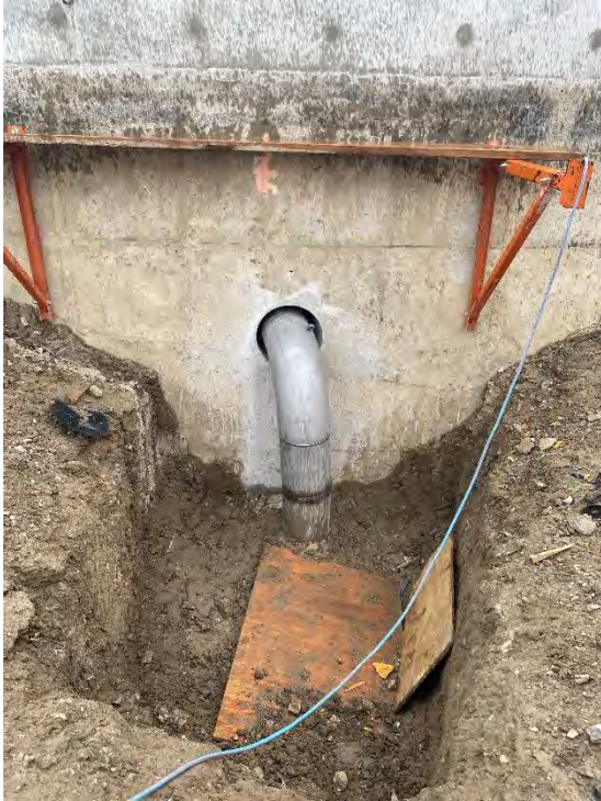
33. DAF No. 1 – Recirculation Piping Through Wall (2022-07-06)
