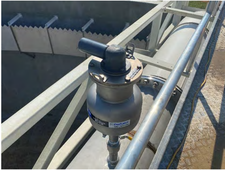
49. DAF No. 1 Influent Piping Air Relief Valve (2022-07-07)
