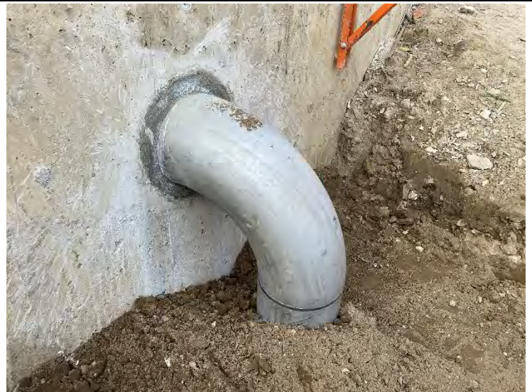
64. DAF No. 1 Recirculation Piping from Tank to Auxiliary Building (2022-07-08)
