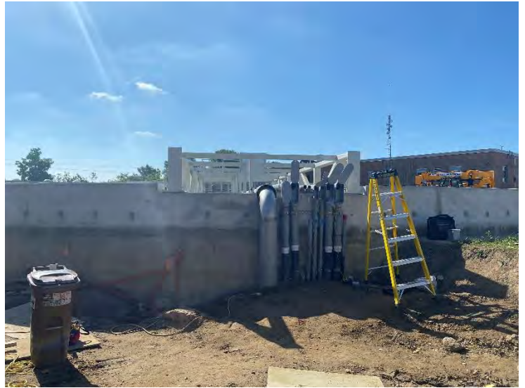
52. DAF No. 1 Tank – Conduit (2022-07-07)
