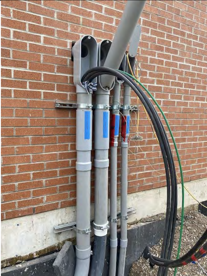
25. Auxiliary Building – 103 mm and 51 mm Conduit through Wall (2022-07-05)
