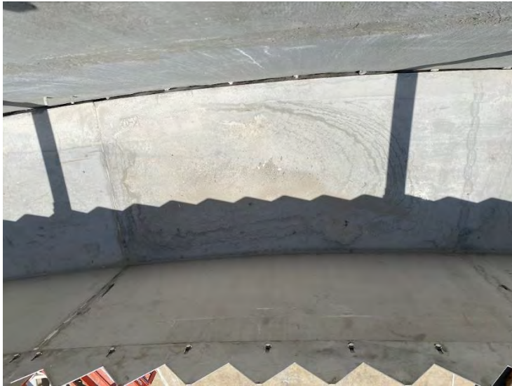
5. DAF No. 1 Effluent Trough – Metal Plate Solution to Fill Gaps (2022-07-04)
