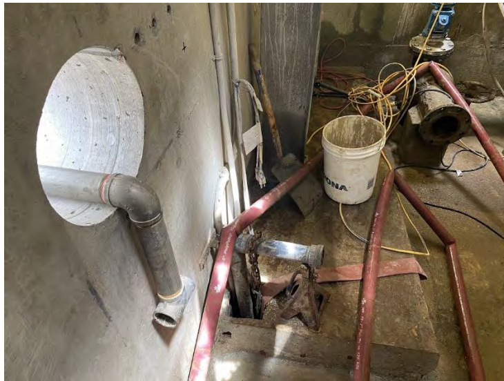
29. DAF No. 1 Blowdown Chamber – Core through Wall for Scum Piping (2022-07-05)
