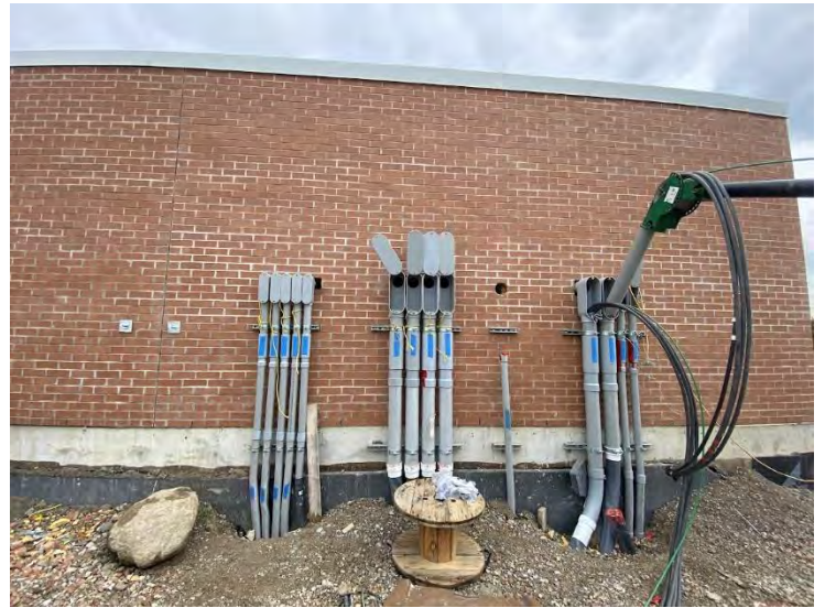
22. Auxiliary Building – Conduit through South Wall (2022-07-05)
