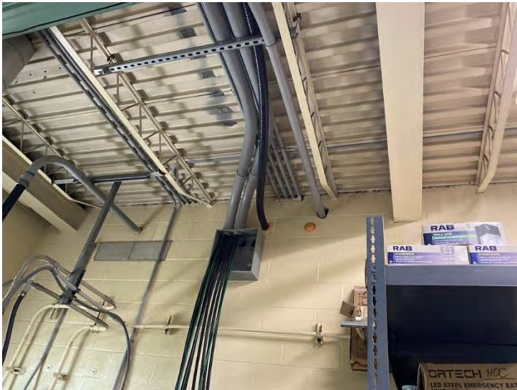
19. Ruthven WTP – Generator Room Conduit for DAF (2022-07-04)
