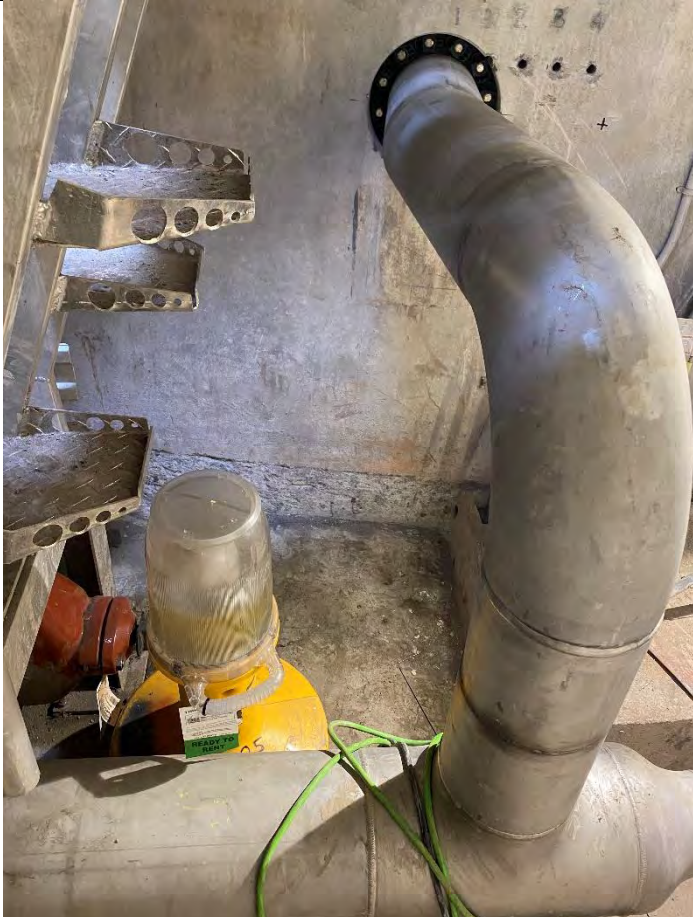
59. DAF No. 1 Blowdown Chamber Scum Piping to Sludge Blowdown Line (2022-07-08)
