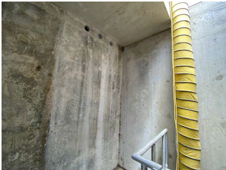
31. DAF No. 1 Blowdown Chamber – Cores Through Wall for Service Water & Conduit (2022-07-05)
