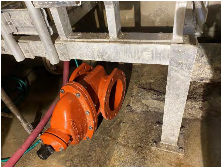
39. DAF No. 1 Blowdown Chamber – Gate Valve for Drain Line (2022-07-07)
