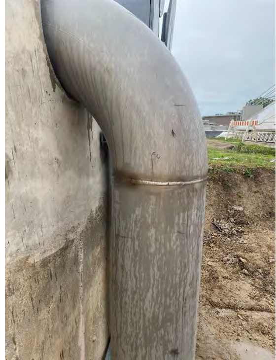
34. DAF No. 1 – Recirculation Piping Through Wall (Weld in progress) (2022-07-06)
