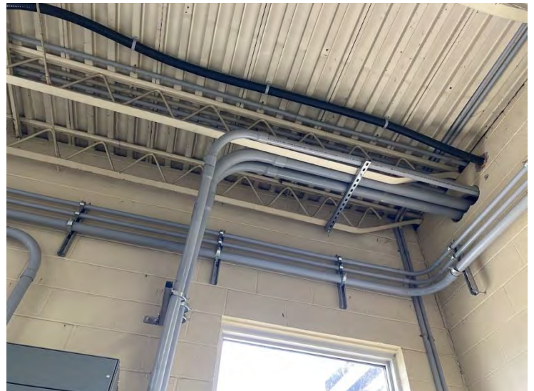
16. Ruthven WTP – CO2 Room Conduit for DAF (2022-07-04)
