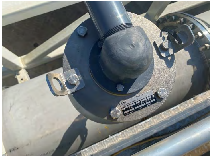
50. DAF No. 1 Influent Piping Air Relief Valve (2022-07-07)
