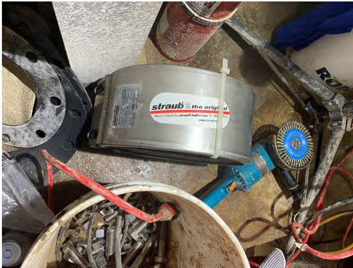
37. DAF No. 1 Blowdown Chamber – Straub Coupling for New Tee Tie-In on Sludge Blowdown Line (2022-07-07)
