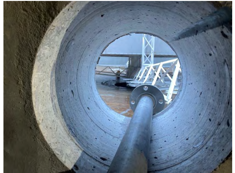
38. DAF No. 1 Blowdown Chamber – Core through Wall for Scum Piping (2022-07-07)
