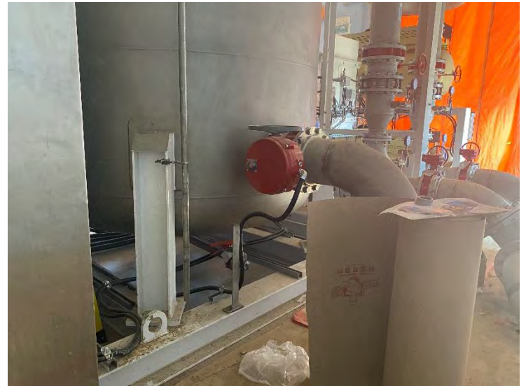
46. Auxiliary Building – Saturation Skid Pressure Relief Valve Drain Piping (to be located further from the power panel) (2022-07-07)
