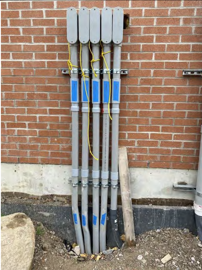
23. Auxiliary Building – 51 mm Conduit through Wall (2022-07-05)
