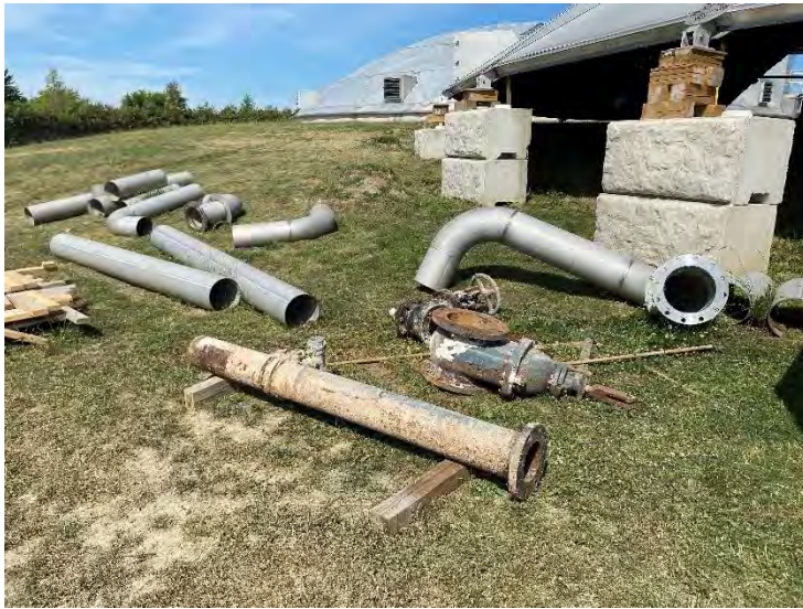
53. Removals from DAF No. 1 Blowdown Chamber (Piping and Valve) (2022-07-07)
