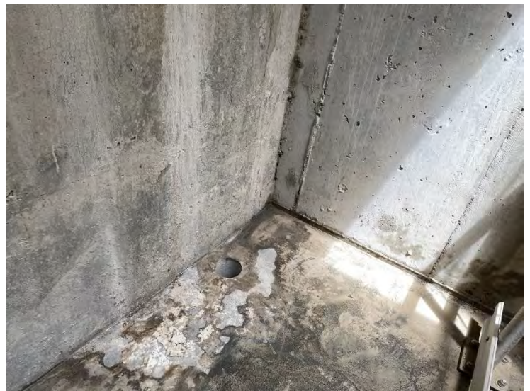
32. DAF No. 1 Blowdown Chamber – Core Through Floor for Service Water (2022-07-05)
