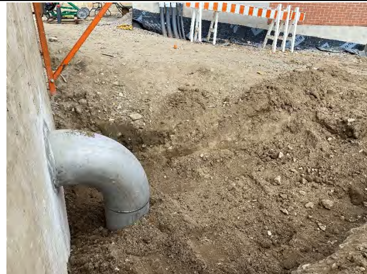
63. DAF No. 1 Recirculation Piping from Tank to Auxiliary Building (2022-07-08)
