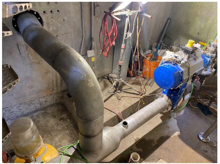
58. DAF No. 1 Blowdown Chamber Scum Piping to Sludge Blowdown Line (2022-07-08)
