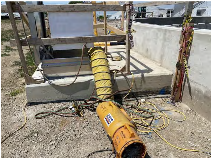
1. DAF No. 1 Blowdown Chamber – Temporary Air Recirculation via Blower for Pipe Removals (2022-07-04)
