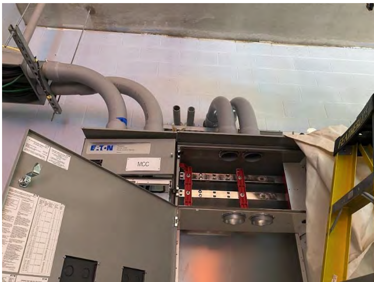
7. Auxiliary Building: MCC Conduit (2022-07-04)
