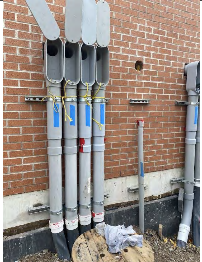
24. Auxiliary Building – 103 mm Conduit through Wall (2022-07-05)
