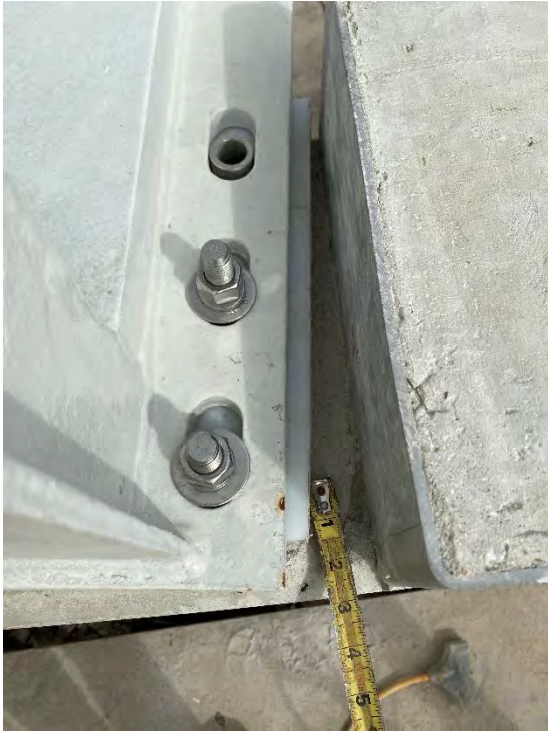
45. DAF No. 1 Bridge Install: Bearing Plates for Bridge Edge Distance (2022-05-25)
