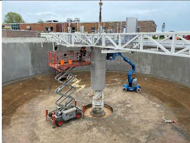
57. DAF No. 1 Equipment Installations (Centre Well) (2022-05-26)
