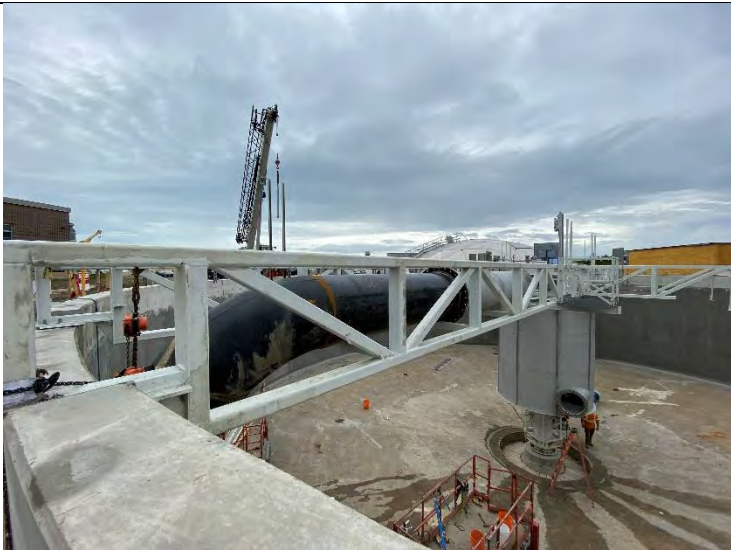
61. DAF No. 1 Equipment Installations (Influent Line) (2022-05-26)
