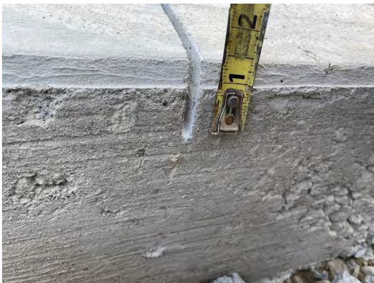
23. Auxiliary Building – Approach Slab Control Joint (2022-05-24)
