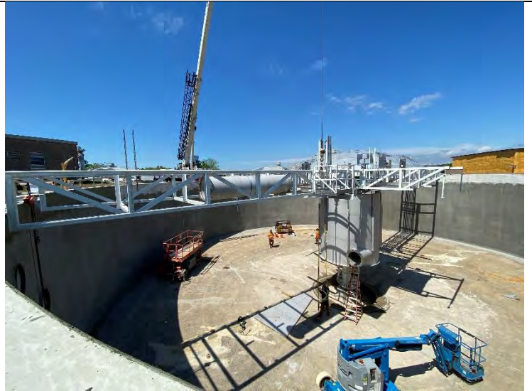
68. DAF No. 1 Tank – Influent Well Installation (2022-05-26)
