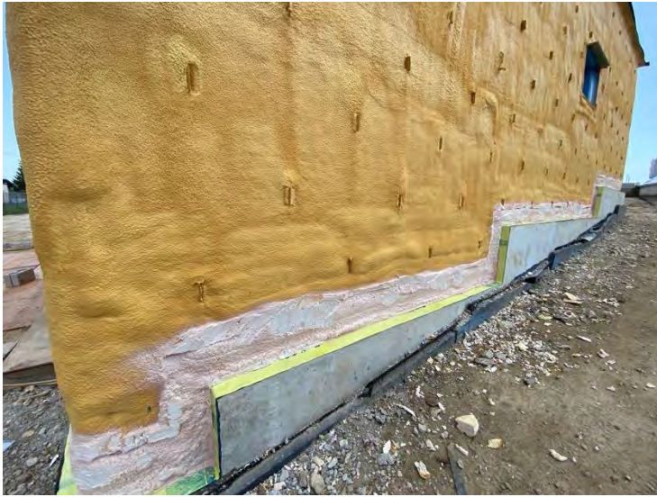
17. Auxiliary Building – Spray Foam Completion (2022-05-24)
