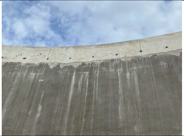
54. DAF No. 1 Tank: Form Ties Removed and Filled (2022-05-25)
