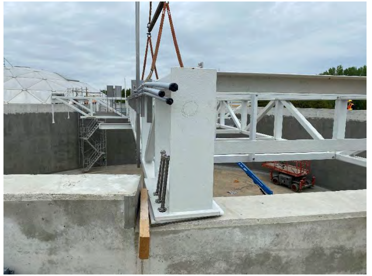
42. DAF No. 1 Bridge Install (2022-05-25)
