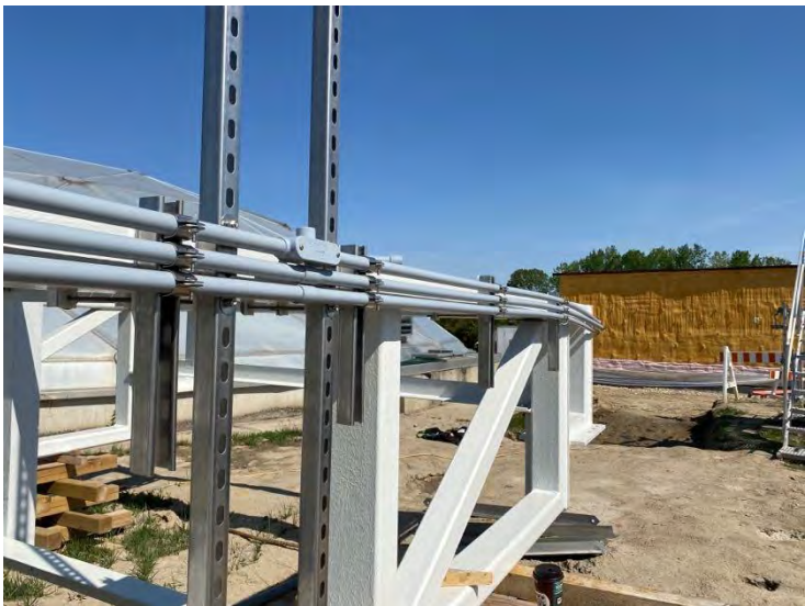
2. DAF No. 1 Bridge with Conduit and Conduit Supports (2022-05-24)
