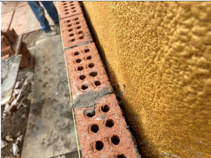
79. Auxiliary Building – Brick Install (2022-05-27)
