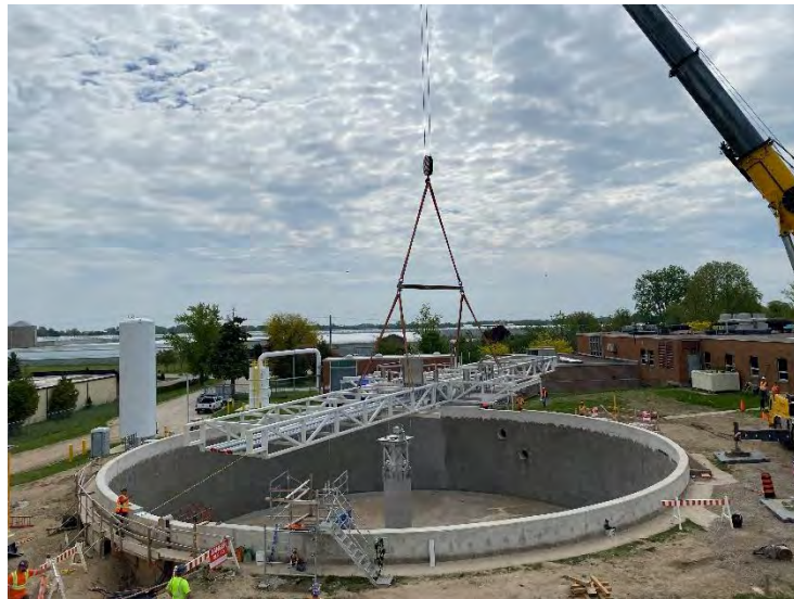
39. DAF No. 1 Bridge Install (2022-05-25)
