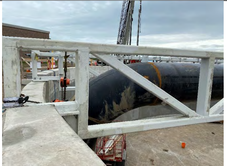
60. DAF No. 1 Equipment Installations (Influent Line) (2022-05-26)
