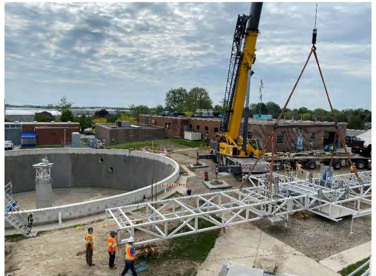
36. DAF No. 1 Bridge Install (2022-05-25)
