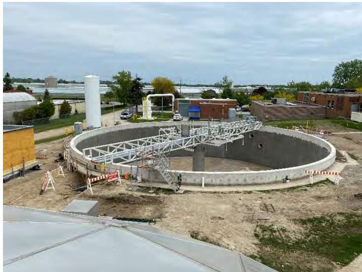
43. DAF No. 1 Bridge Install (2022-05-25)
