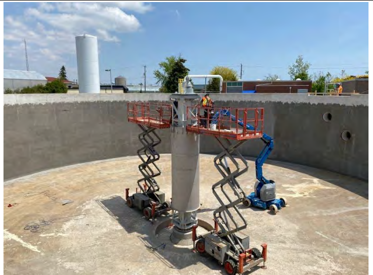
20. DAF No. 1 – Corrections to Centre Cage due to Interference from Centre Cage / Drive Interference (2022-05-24)
