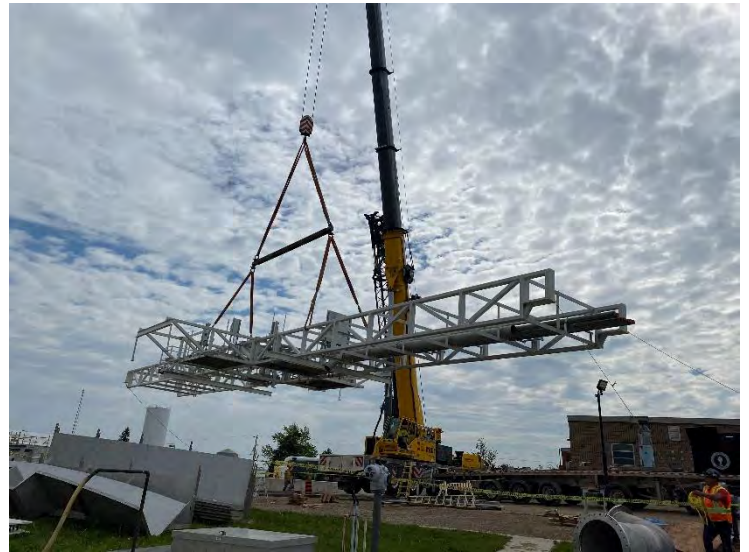
38. DAF No. 1 Bridge Install (2022-05-25)
