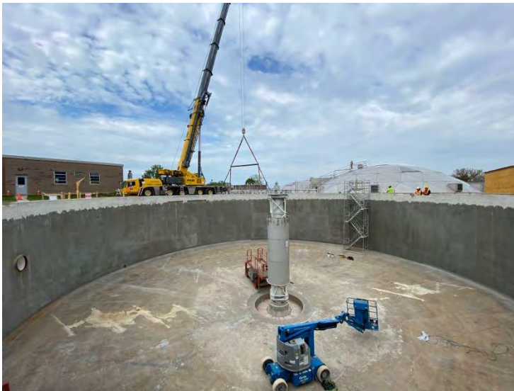
33. DAF No. 1 Bridge Install (2022-05-25)
