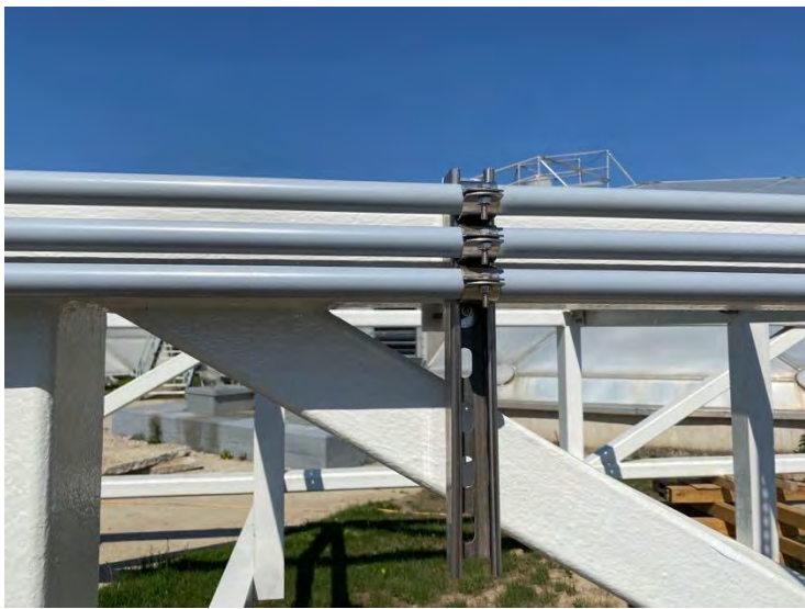
3. DAF No. 1 Bridge with Conduit and Conduit Supports (2022-05-24)
