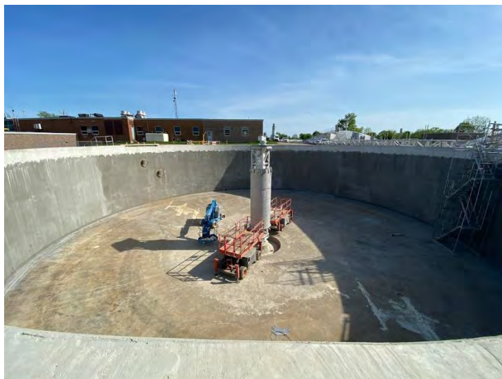
25. DAF No. 1 – Centre Cage and Column (2022-05-24)
