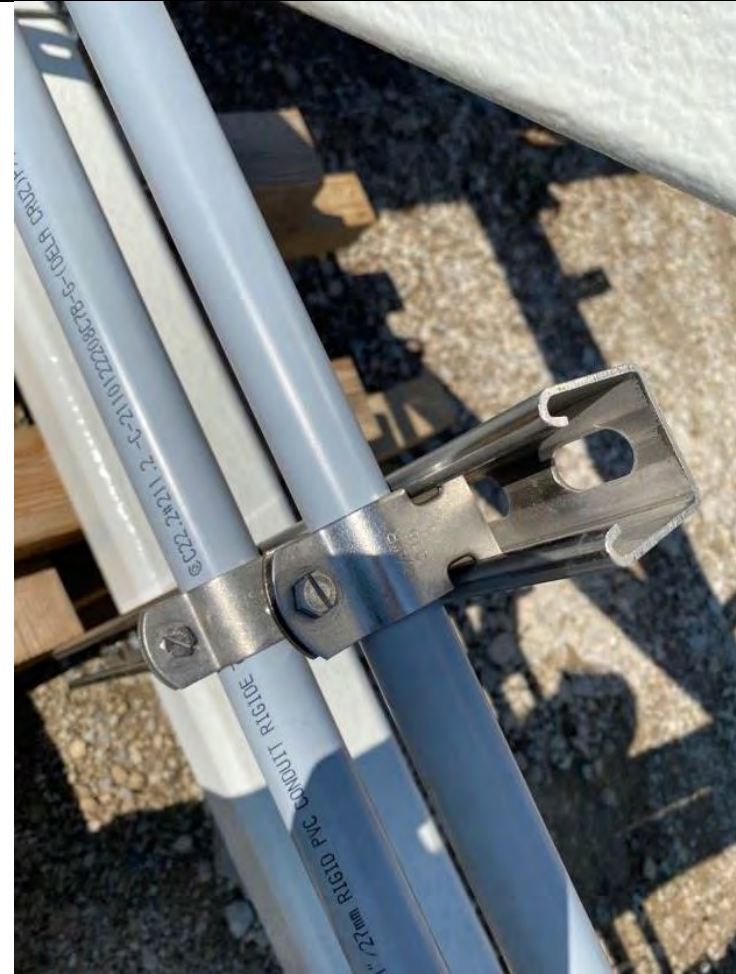
9. DAF No. 1 Bridge with Conduit and Conduit Supports (2022-05-24)
