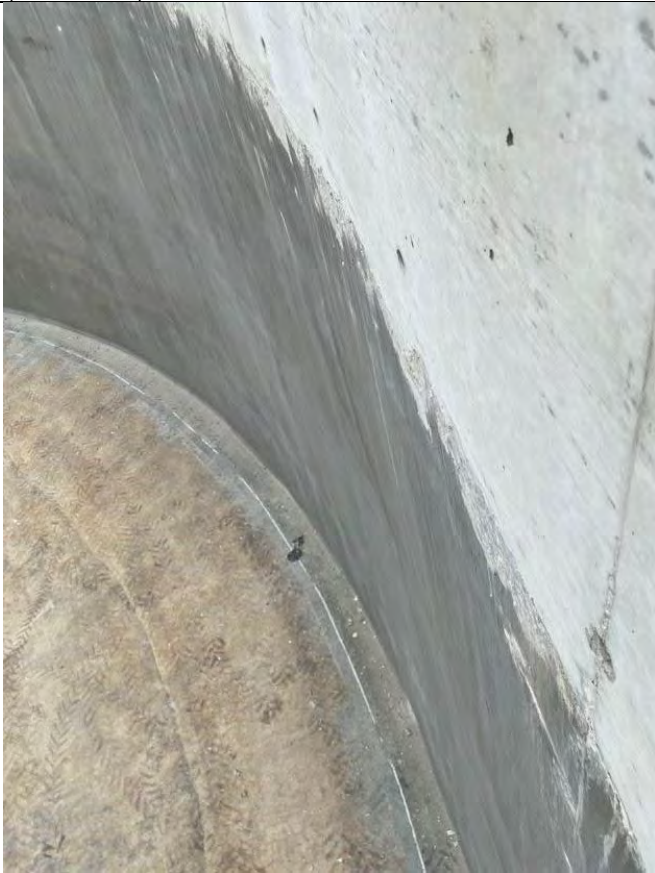
32. DAF No. 1 – Removal of Form Ties (2022-05-25)
