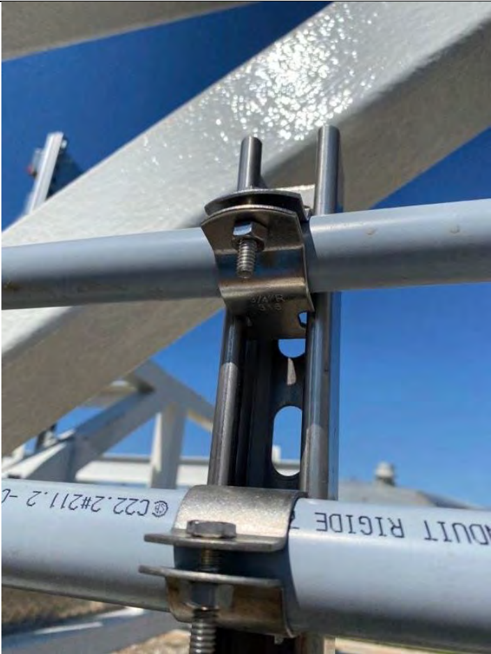
8. DAF No. 1 Bridge with Conduit and Conduit Supports (2022-05-24)
