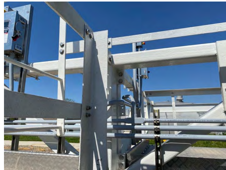
11. DAF No. 1 Bridge with Conduit and Conduit Supports (2022-05-24)
