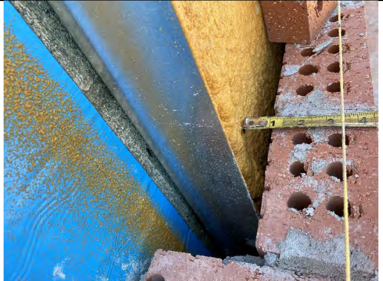
82. Auxiliary Building – Brick Install Air Gap of 1" (2022-05-27)
