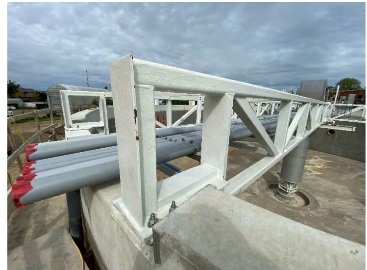
44. DAF No. 1 Bridge Install (2022-05-25)
