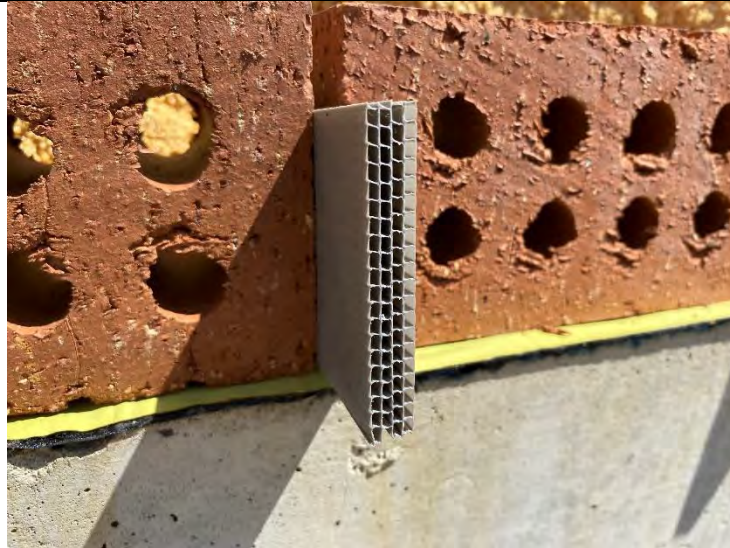
83. Auxiliary Building: Cell Vent Example (2022-05-27)
