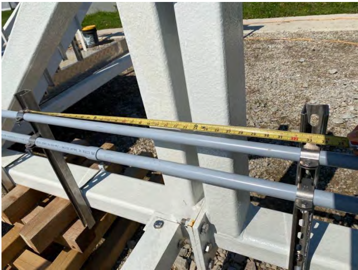
6. DAF No. 1 Bridge with Conduit and Conduit Supports (2022-05-24)
