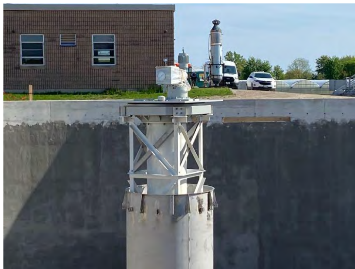
26. DAF No. 1 – Centre Cage and Column: Cage and Drive Interference Corrected (2022-05-24)
