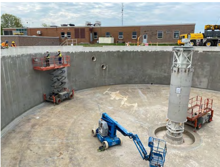
29. DAF No. 1 – Removal of Form Ties and Fill in Form Tie Holes (2022-05-25)
