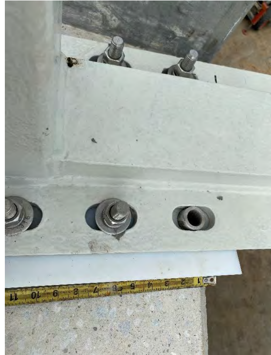
46. DAF No. 1 Bridge Install: Bearing Plates for Bridge Edge Distance (2022-05-25)
