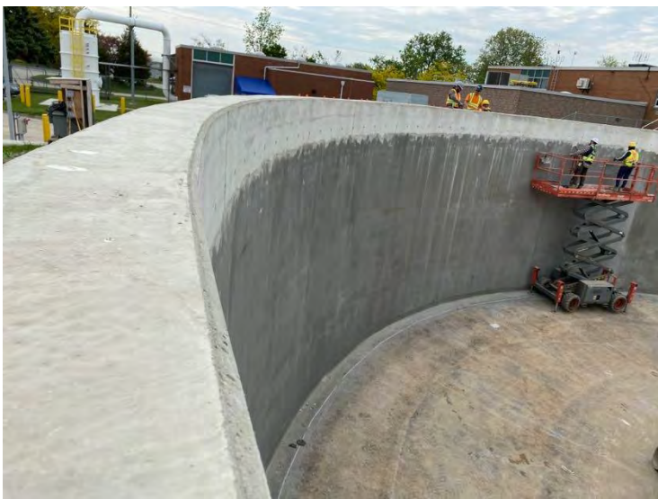
30. DAF No. 1 – Removal of Form Ties and Fill in Form Tie Holes (2022-05-25)
