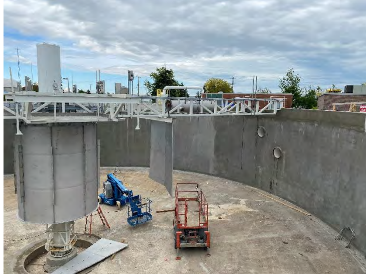
73. DAF No. 1 – Center Well (11.5m) Installation (2022-05-27)
