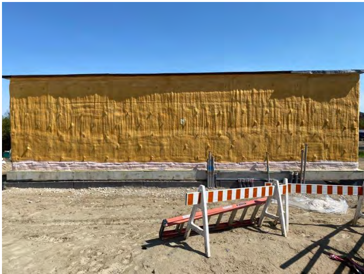
13. Auxiliary Building – Spray Foam Completion (2022-05-24)
