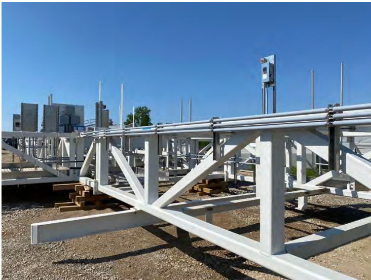
5. DAF No. 1 Bridge with Conduit and Conduit Supports (2022-05-24)
