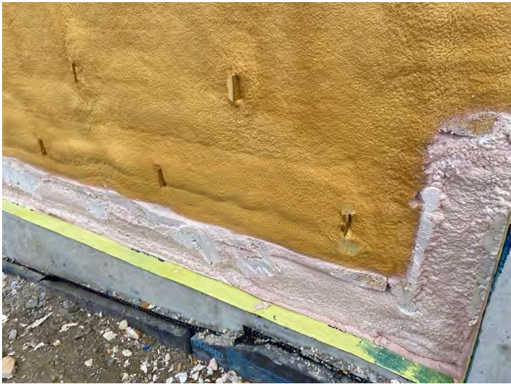
16. Auxiliary Building – Spray Foam Completion (2022-05-24)
