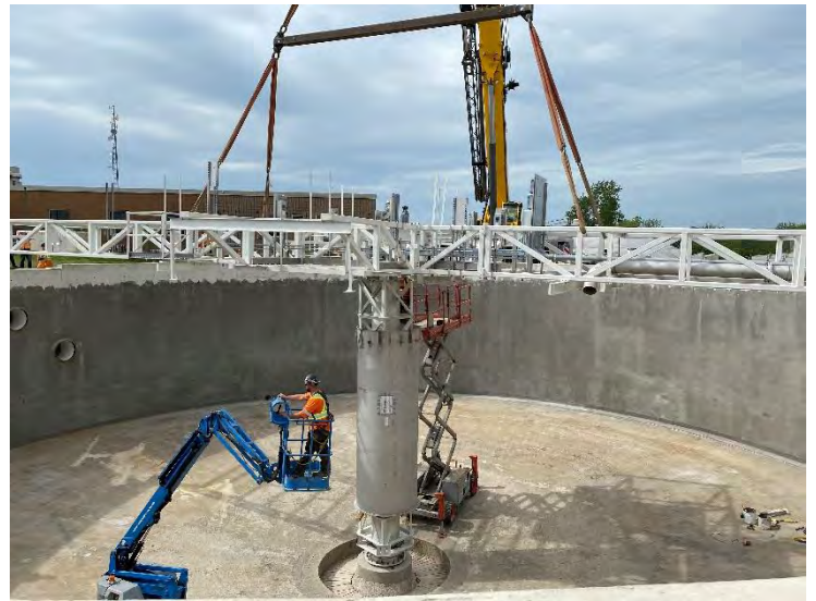
40. DAF No. 1 Bridge Install (2022-05-25)
