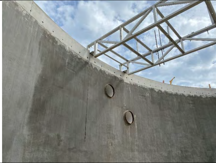
53. DAF No. 1 Tank: Form Ties Removed and Filled (2022-05-25)
