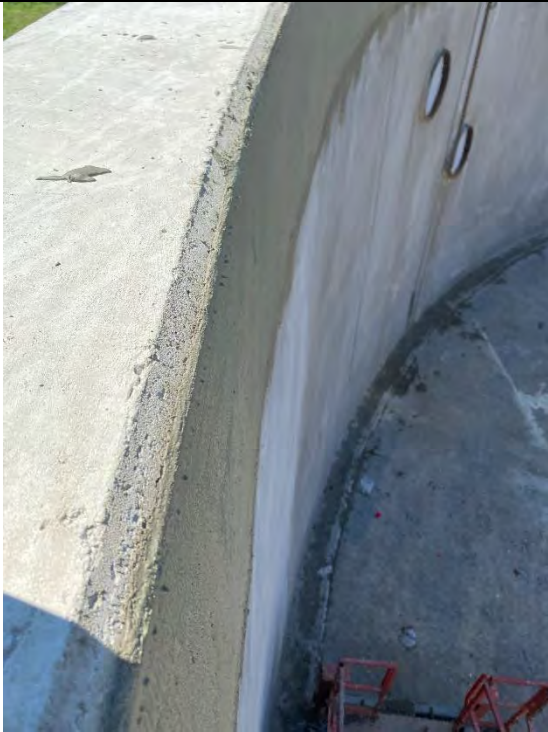
69. DAF No. 1 Tank – Coatings on Wall Extension (2022-05-26)
