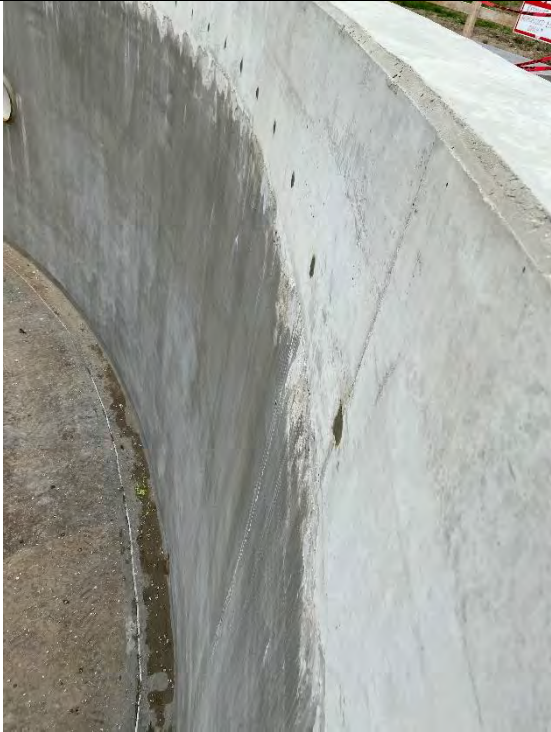
52. DAF No. 1 Tank: Form Ties Removed and Filled (2022-05-25)
