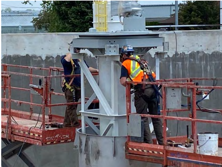
21. DAF No. 1 – Corrections to Centre Cage due to Interference from Centre Cage / Drive Interference (2022-05-24)
