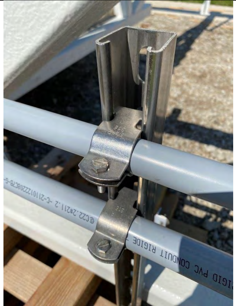
10. DAF No. 1 Bridge with Conduit and Conduit Supports (2022-05-24)
