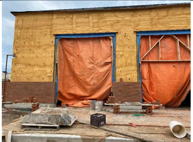
84. Auxiliary Building: Brick Install (2022-05-27)
