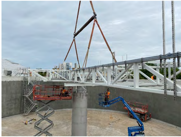
41. DAF No. 1 Bridge Install (2022-05-25)
