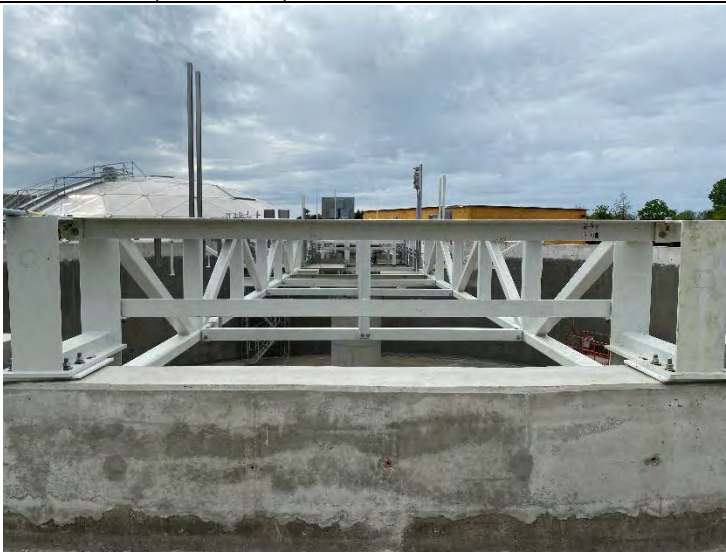
47. DAF No. 1 Bridge Install (2022-05-25)
