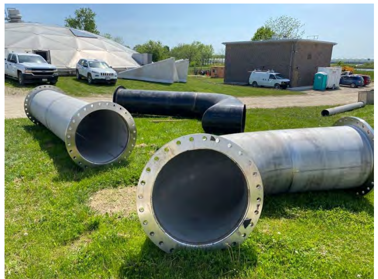
24. DAF No. 1 Influent and Effluent Piping (750mm) (2022-05-24)
