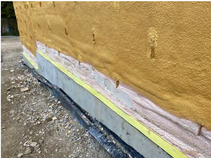
14. Auxiliary Building – Spray Foam Completion (2022-05-24)
