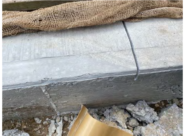
22. Auxiliary Building – Approach Slab Control Joint (2022-05-24)
