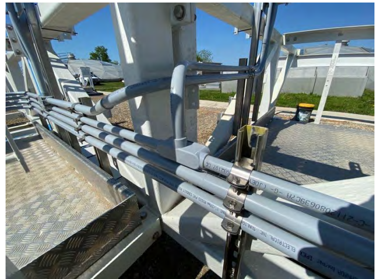
12. DAF No. 1 Bridge with Conduit and Conduit Supports (2022-05-24)
