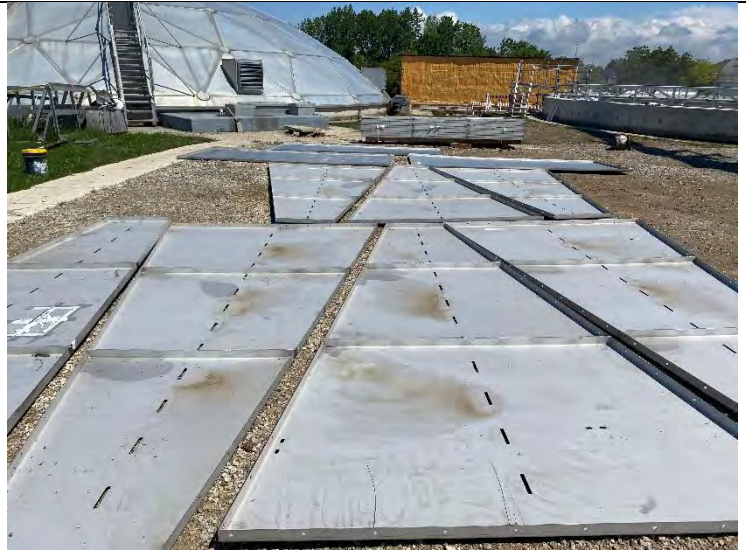
72. DAF No. 1 Tank – Center Well Pieces (11.5m) (2022-05-26)
