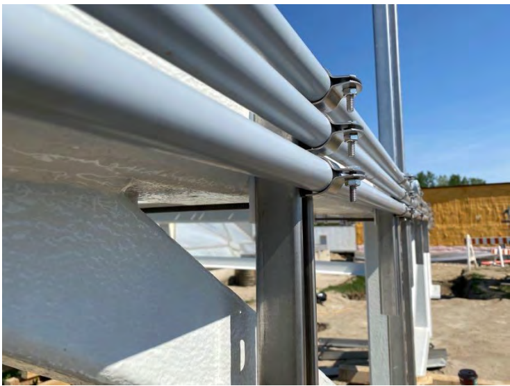
4. DAF No. 1 Bridge with Conduit and Conduit Supports (2022-05-24)
