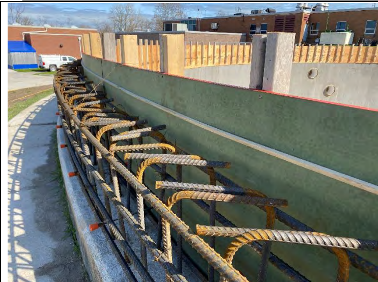
53. DAF No. 1 Tank – Interior Formply Chamfer Strip (2022-05-04)
