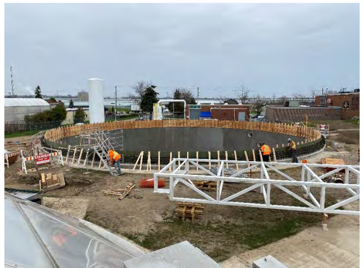
24. DAF No. 1 Tank – Interior Forms and Support and Form ties (2022-05-03)
