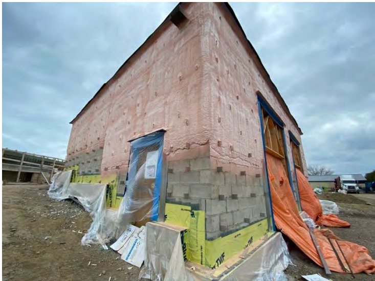
15. Auxiliary Building – Spray Foam Insulation (2022-05-02)
