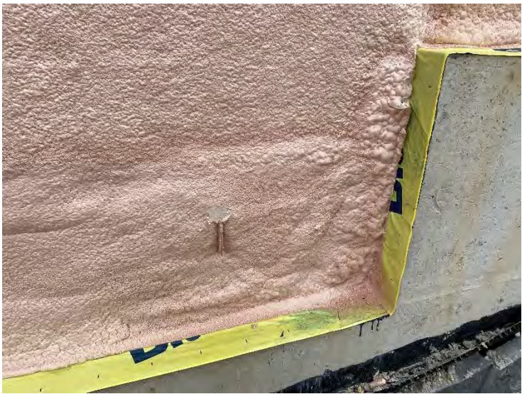
74. Auxiliary Building – Spray Foam and Vapour Barrier Intersection / Overlap (2022-05-05)
