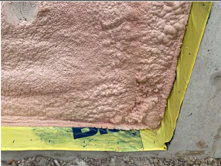
72. Auxiliary Building – Spray Foam and Vapour Barrier Intersection / Overlap (2022-05-05)
