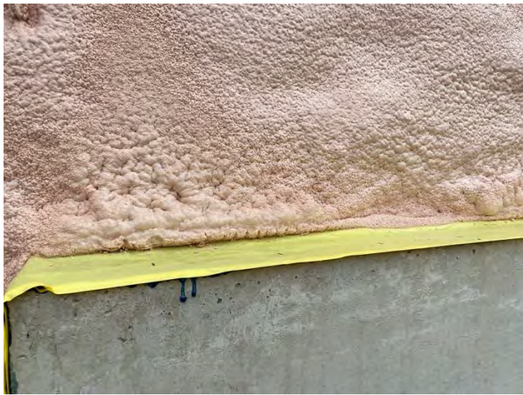
73. Auxiliary Building – Spray Foam and Vapour Barrier Intersection / Overlap (2022-05-05)
