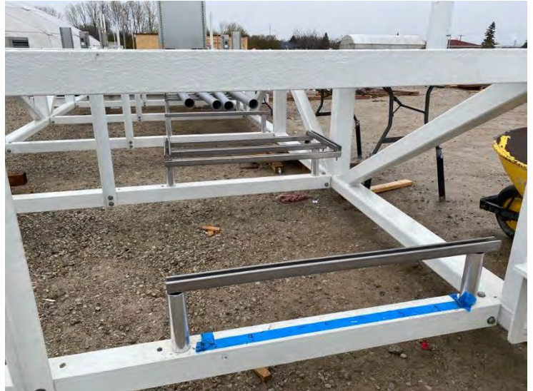
80. DAF No. 1 Bridge – Conduit Supports (2022-05-06)
