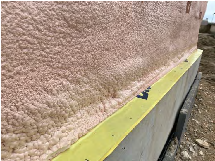
75. Auxiliary Building – Spray Foam and Vapour Barrier Intersection / Overlap (2022-05-05)
