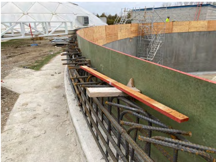
2. DAF No. 1 Tank – Interior Form (2022-05-02)
