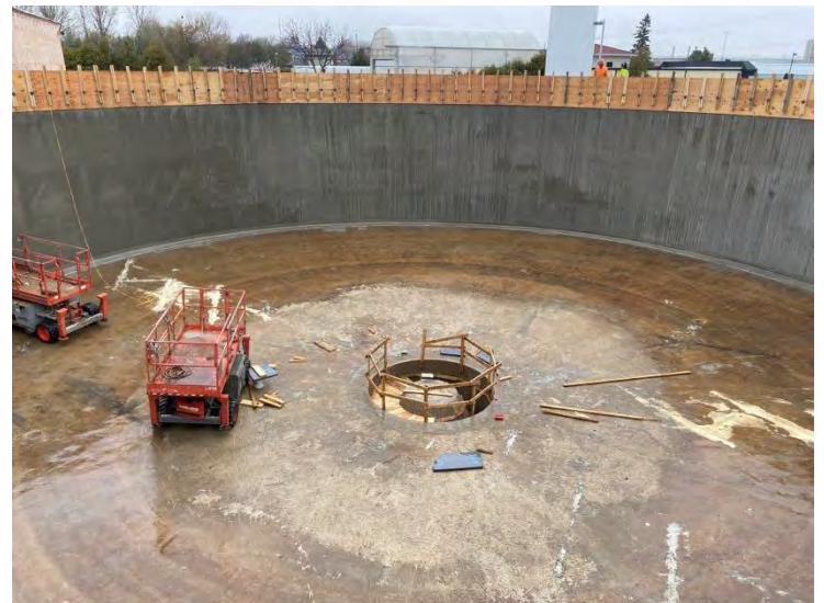
28. DAF No. 1 Tank – Interior Forms and Supports (2022-05-03)
