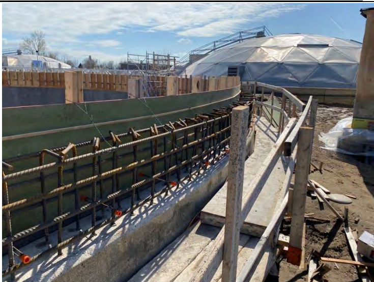
54. DAF No. 1 Tank – Interior Formply Chamfer Strip (2022-05-04)
