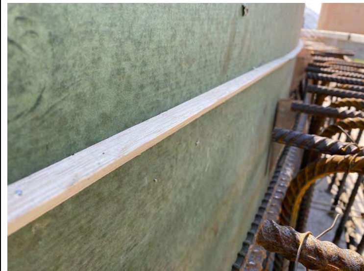
55. DAF No. 1 Tank – Interior Formply Chamfer Strip (2022-05-04)
