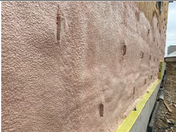
71. Auxiliary Building – Spray Foam and Vapour Barrier Intersection / Overlap (2022-05-05)
