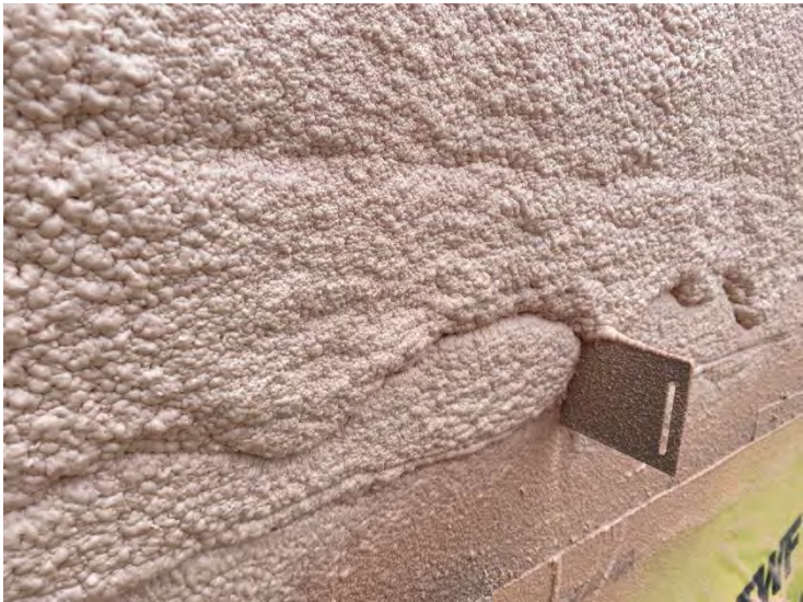
18. Auxiliary Building – Spray Foam Insulation (2022-05-02)
