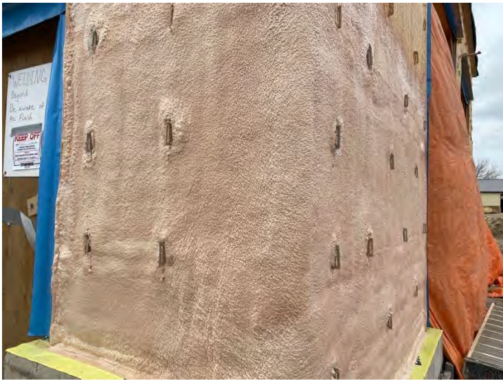
68. Auxiliary Building – Spray Foam (2022-05-05)
