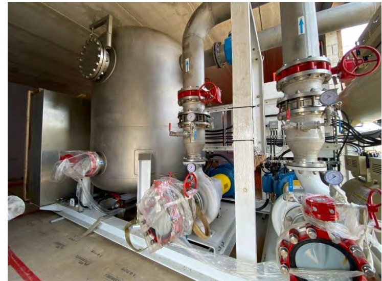
48. DAF No. 1 Saturation Skid (2022-05-04)
