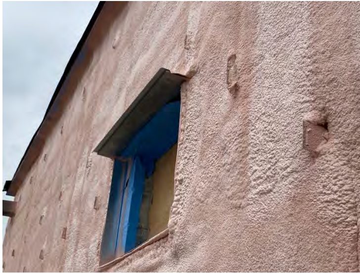
21. Auxiliary Building – Spray Foam Insulation (2022-05-02)
