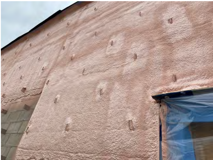
16. Auxiliary Building – Spray Foam Insulation (2022-05-02)
