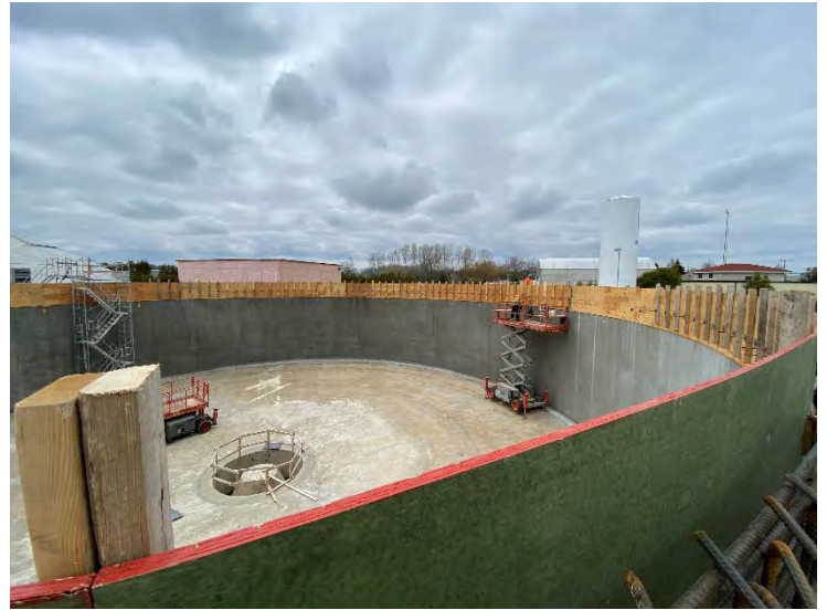
22. DAF No. 1 Tank – Interior Forms and Support (2022-05-02)
