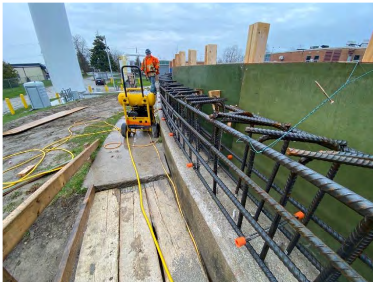
27. DAF No. 1 Tank – Interior Forms and Form Ties (2022-05-03)
