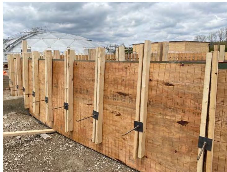
60. DAF No. 1 Tank – Exterior Form (2022-05-05)
