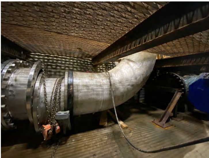
51. Valve Room – DAF No. 1 Influent Line Pipe Spool and Gasket for Victaulic Coupling (2022-05-04)
