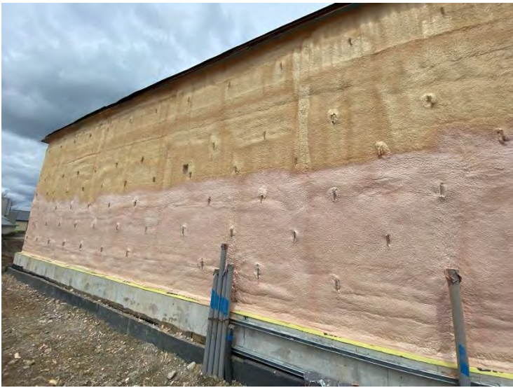
66. Auxiliary Building – Spray Foam (2022-05-05)
