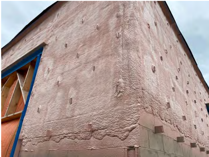
13. Auxiliary Building – Spray Foam Insulation (2022-05-02)
