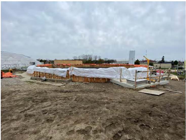
76. DAF No. 1 Tank – Walls Tarped (2022-05-05)
