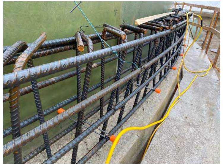
26. DAF No. 1 Tank – Interior Forms and Form Ties (2022-05-03)
