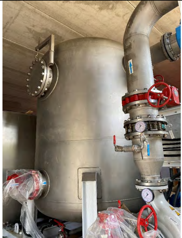
50. DAF No. 1 Saturation Skid (2022-05-04)
