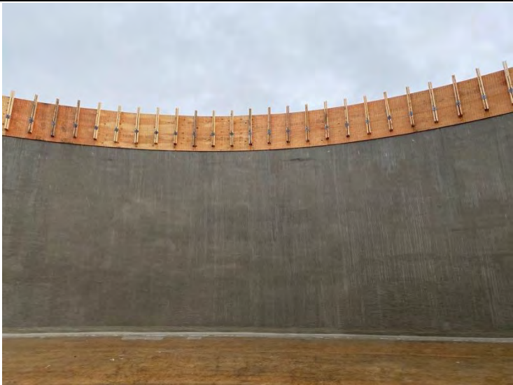
35. DAF No. 1 Tank – Interior Forms (2022-05-03)
