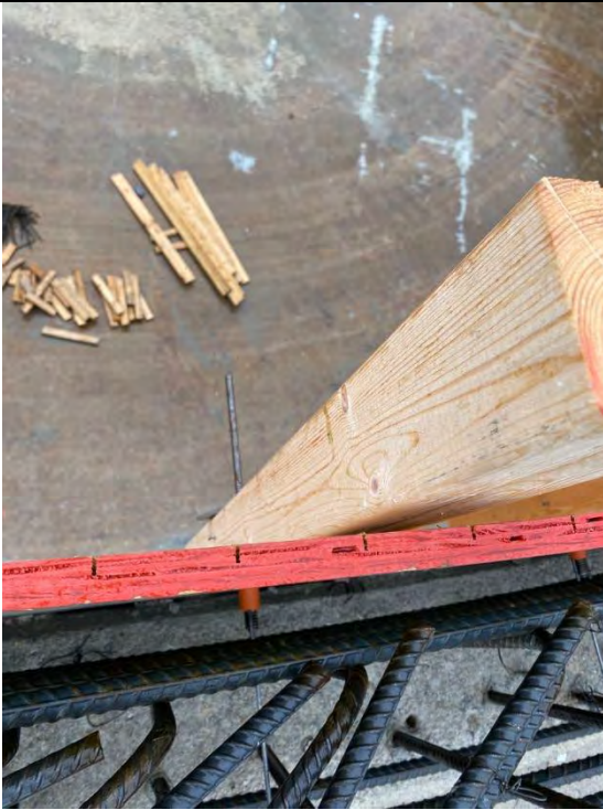
29. DAF No. 1 Tank – Interior Forms and Supports with Form tie (2022-05-03)
