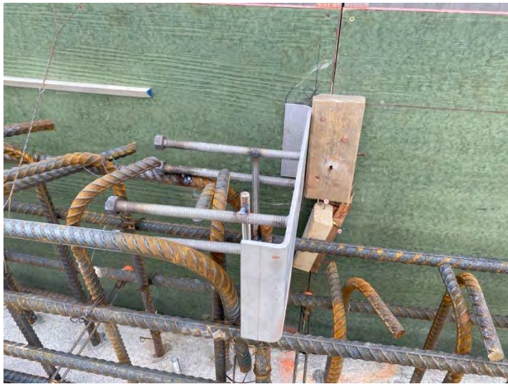
77. DAF No. 1 Tank – Bent Plate with Nelson Studs Welded and Attached to Rebar (2022-05-05)
