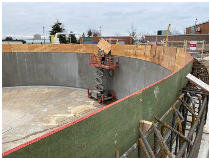
3. DAF No. 1 Tank – Interior Form (2022-05-02)
