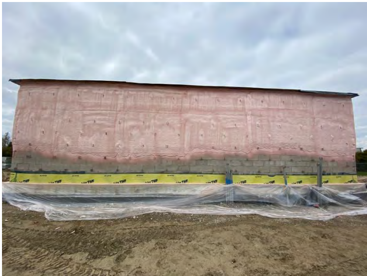
19. Auxiliary Building – Spray Foam Insulation (2022-05-02)
