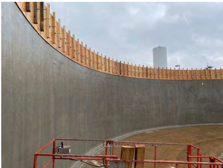
33. DAF No. 1 Tank – Interior Forms (2022-05-03)
