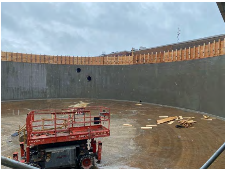
34. DAF No. 1 Tank – Interior Forms (2022-05-03)
