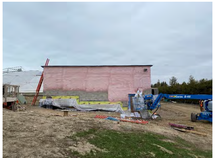
12. Auxiliary Building – Spray Foam Insulation (2022-05-02)
