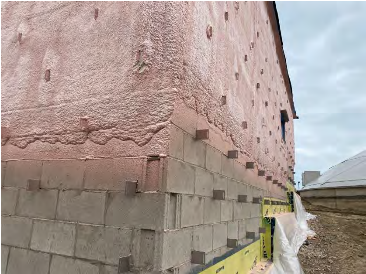
14. Auxiliary Building – Spray Foam Insulation (2022-05-02)
