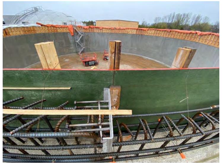
82. DAF No. 1 Tank – Bent Plate for Bridge and Dome Edge(2022-05-06)
