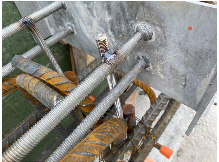
78. DAF No. 1 Tank – Bent Plate with Nelson Studs Welded and Attached to Rebar (2022-05-05)
