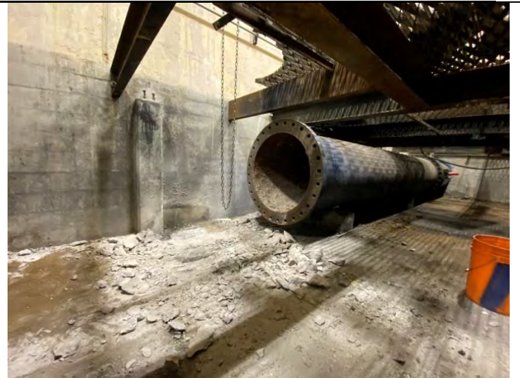
38. Valve Room – West Tee Removed and Concrete Support Chipped Away (2022-02-02)
