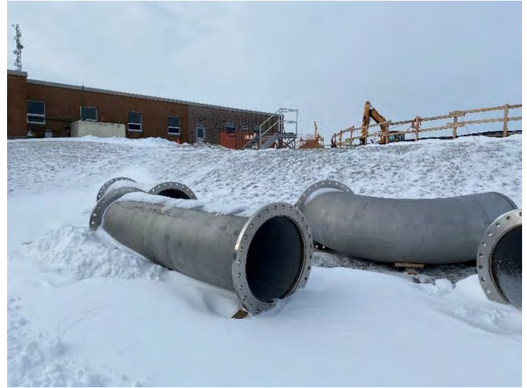
46. Valve Room – Process Piping for DAF No. 1 Influent Line (2022-02-04)
