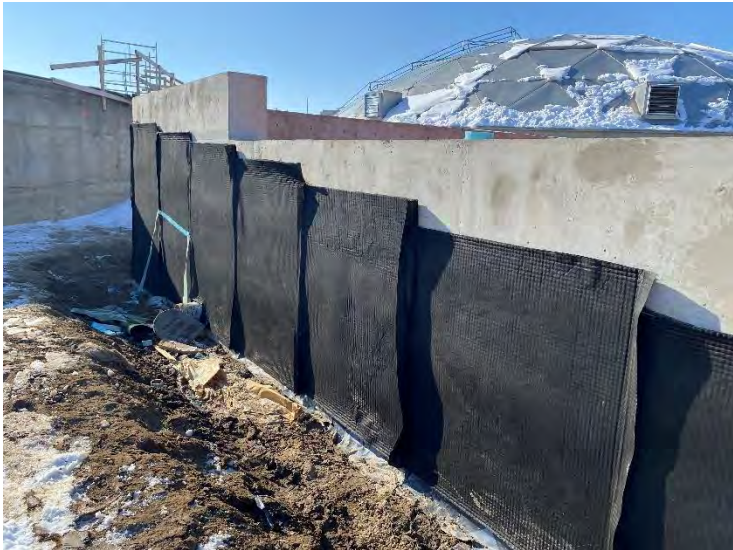
7. Auxiliary Building – Hydroduct 220 Drainage Sheet (2022-01-31)
