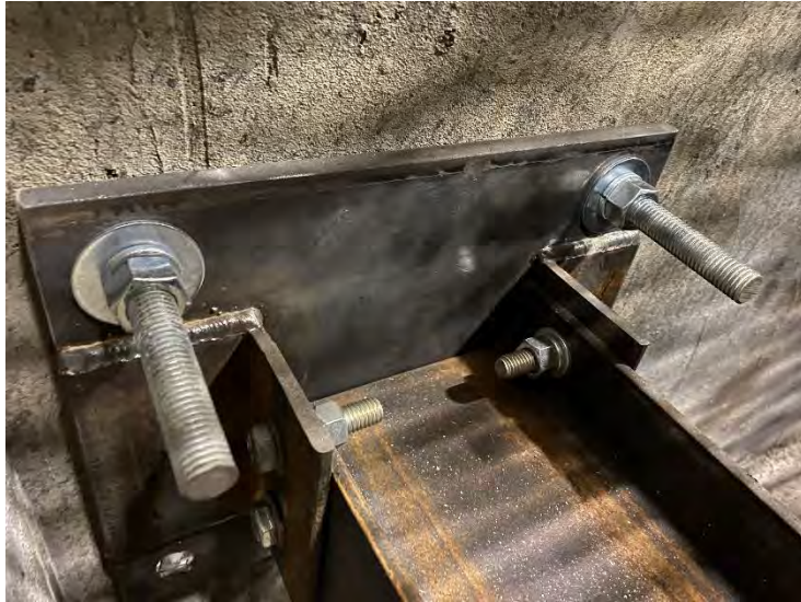
45. Valve Room East Tee Blind Flange – Restraint in Progress (2022-02-03)
