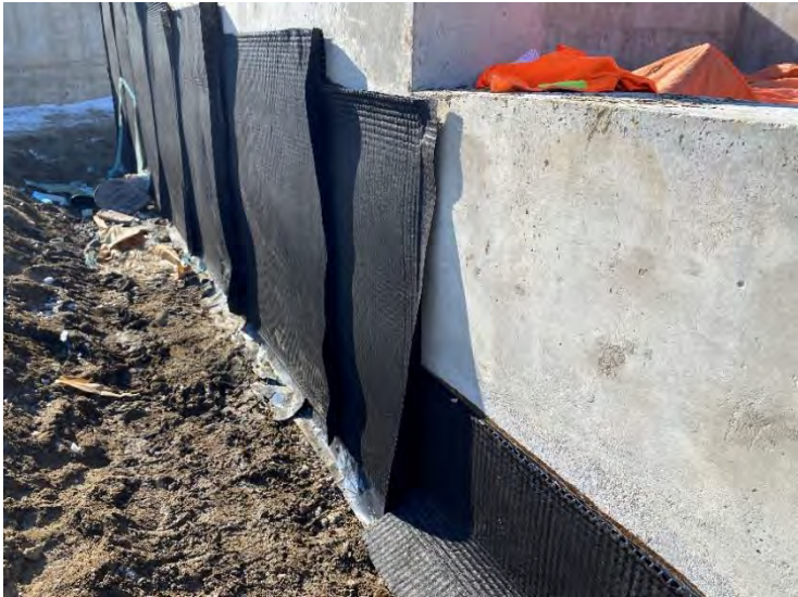
8. Auxiliary Building – Hydroduct 220 Drainage Sheet (2022-01-31)
