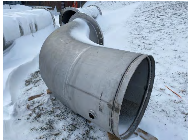
48. Valve Room – Process Piping for DAF No. 1 Influent Line (2022-02-04)
