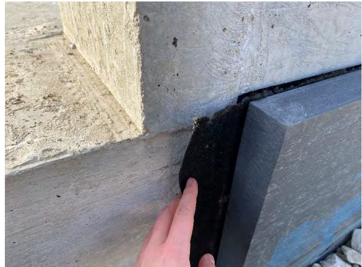
24. Auxiliary Building – Insulation Installation (Styrofoam Highload 40) (2022-02-01)
