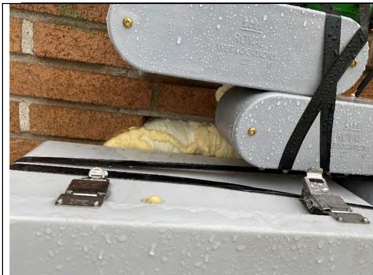
29. Fire Stop on Electrical Pull Box on North Side of WTP (2022-02-02)
