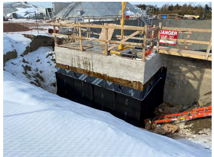
26. Blowdown Chamber – Waterproofing System Installation (2022-02-01)
