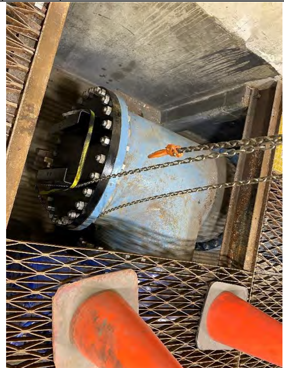
40. Valve Room – Blind Flange Installed (2022-02-03)
