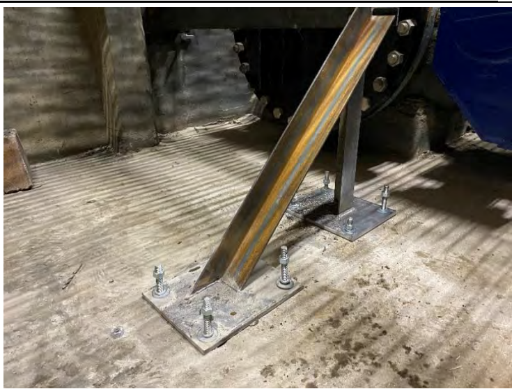
54. Valve Room – Restrained East Tee A Frame (2022-02-04)
