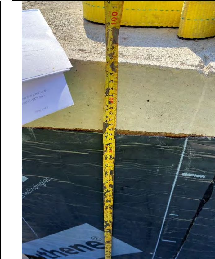
5. Auxiliary Building – Waterproofing Membrane (Bituthene 3000) (2022-01-31)
