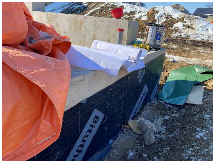
1. Auxiliary Building – Waterproofing Membrane (Bituthene 3000) (2022-01-31)
