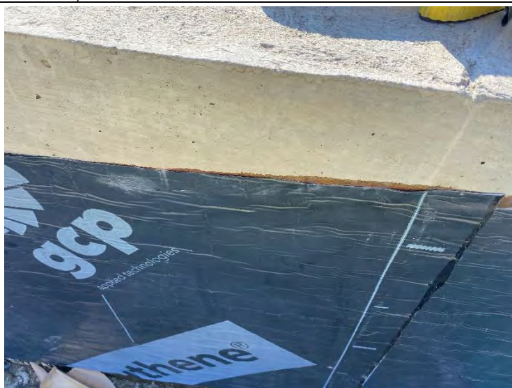
3. Auxiliary Building – Waterproofing Membrane (Bituthene 3000) (2022-01-31)
