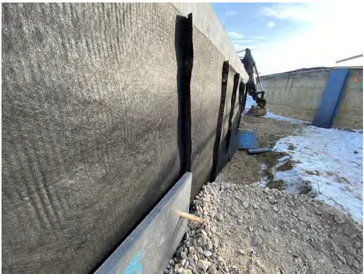
23. Auxiliary Building – Insulation Installation (Styrofoam Highload 40) (2022-02-01)
