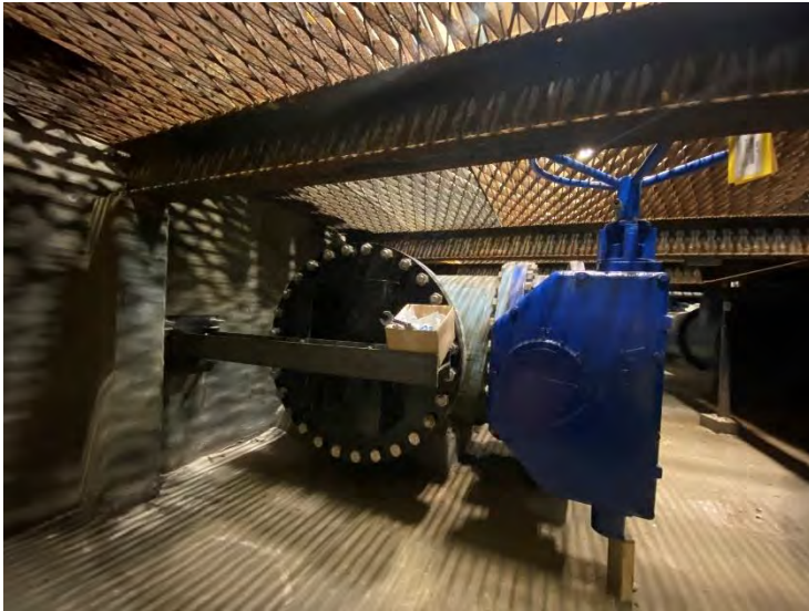
43. Valve Room East Tee Blind Flange – Restraint in Progress (2022-02-03)
