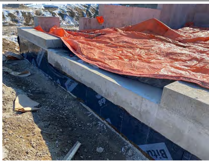
4. Auxiliary Building – Waterproofing Membrane (Bituthene 3000) (2022-01-31)
