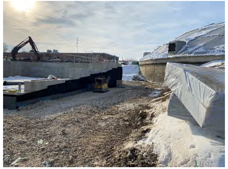
22. Auxiliary Building – Insulation Installation (Styrofoam Highload 40) (2022-02-01)
