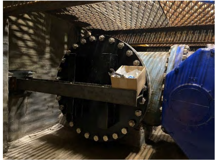
44. Valve Room East Tee Blind Flange – Restraint in Progress (2022-02-03)
