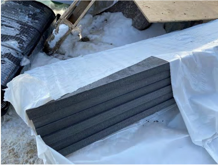
21. Auxiliary Building – Insulation (Styrofoam Highload 40) (2022-02-01)
