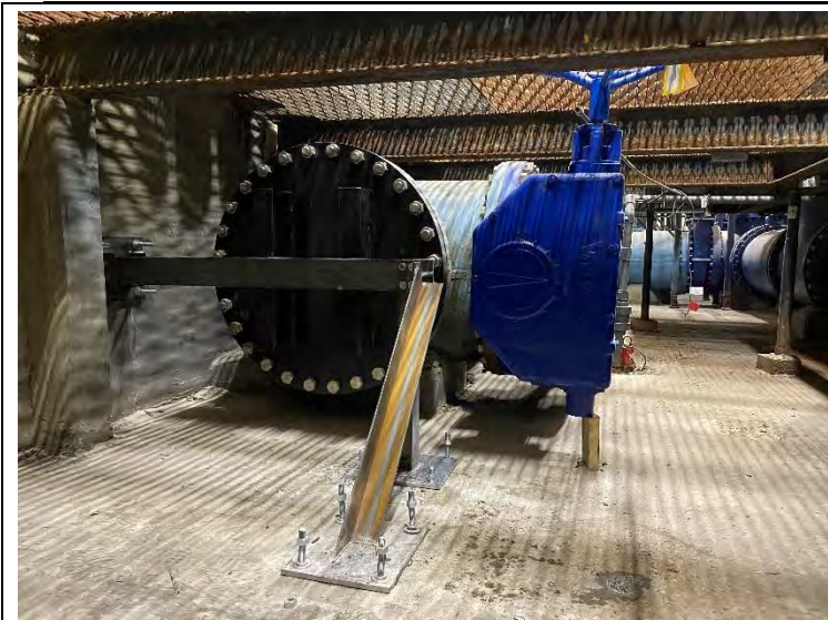
53. Valve Room – Restrained East Tee in Progress (2022-02-04)
