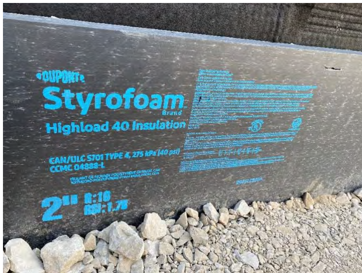
25. Auxiliary Building – Insulation Installation (Styrofoam Highload 40) (2022-02-01)
