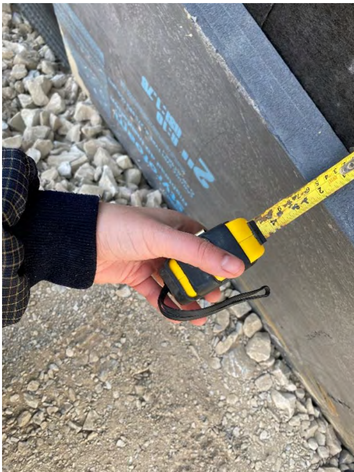
19. Auxiliary Building – Insulation Installation (Styrofoam Highload 40) (2022-02-01)
