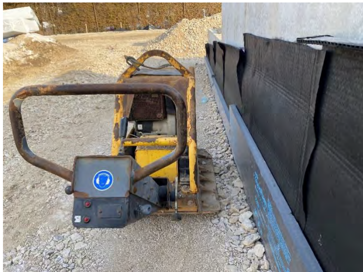
17. Auxiliary Building – Granular B-2 Compaction (2022-02-01)
