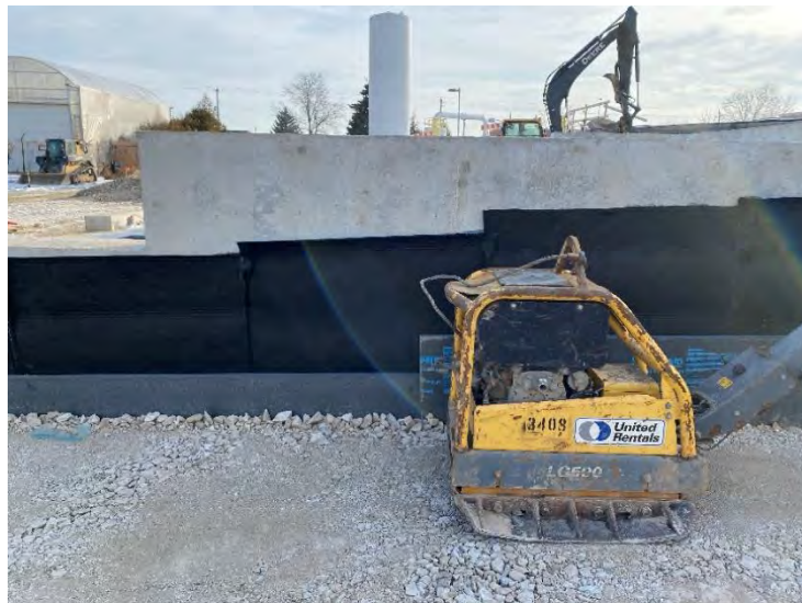
18. Auxiliary Building – Granular B-2 Compaction (2022-02-01)
