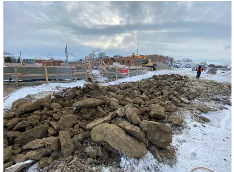
52. Frost Ripping South of Auxiliary Building for Water Service Line (2022-02-04)
