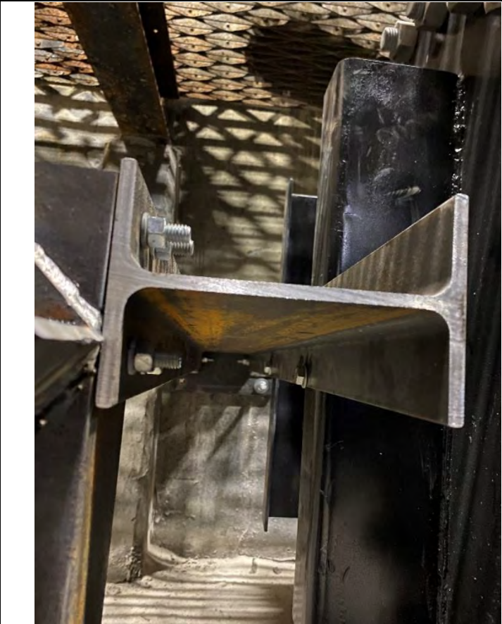
58. Valve Room – Restrained East Tee W Beam (2022-02-04)
