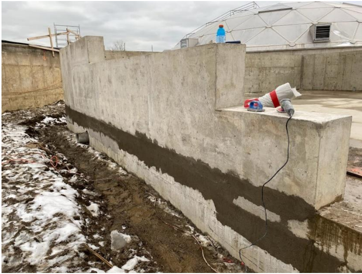
19. Auxiliary Building – Wall Pre Waterproofing & Masonry Repairs in Progress (2022-01-05)
