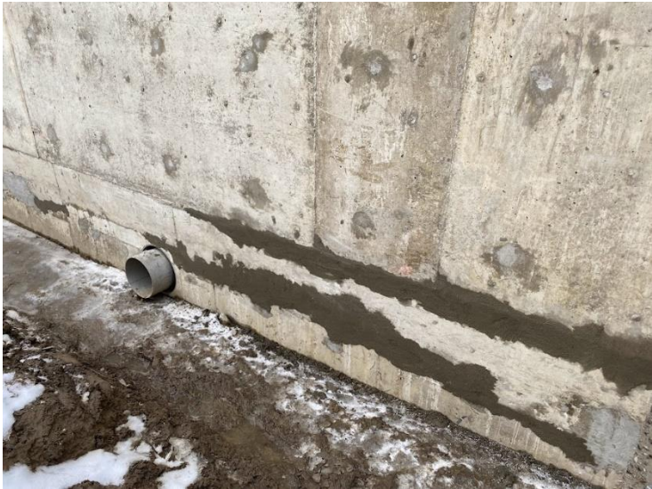
15. Auxiliary Building – Wall Pre Waterproofing & Masonry Repairs in Progress (2022-01-05)
