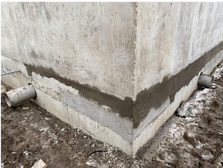
17. Auxiliary Building – Wall Pre Waterproofing & Masonry Repairs in Progress (2022-01-05)
