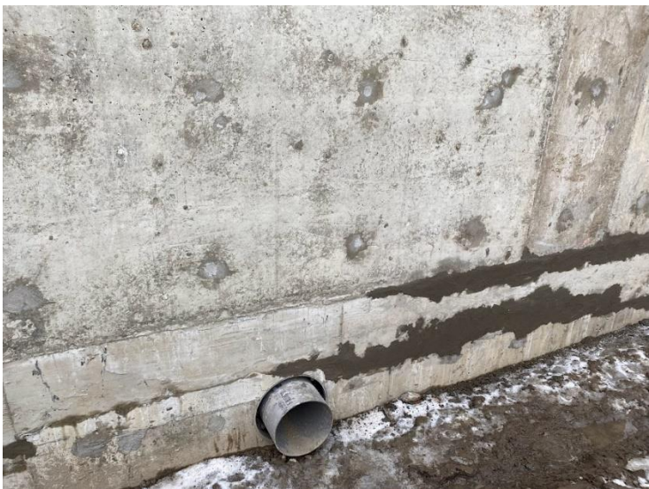
14. Auxiliary Building – Wall Pre Waterproofing & Masonry Repairs in Progress (2022-01-05)
