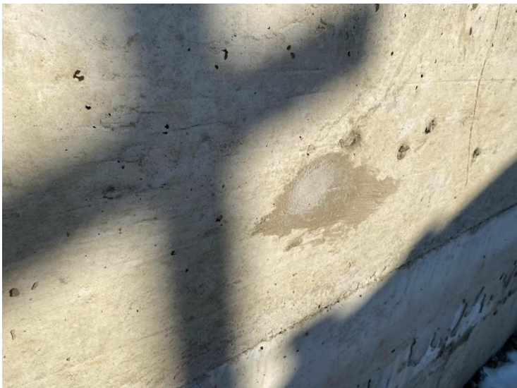
6. Auxiliary Building – Wall Pre Waterproofing & Masonry Repairs in Progress (2022-01-04)
