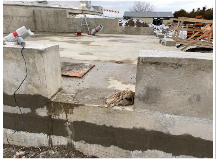
20. Auxiliary Building – Wall Pre Waterproofing & Masonry Repairs in Progress (East Door Access) (2022-01-05)
