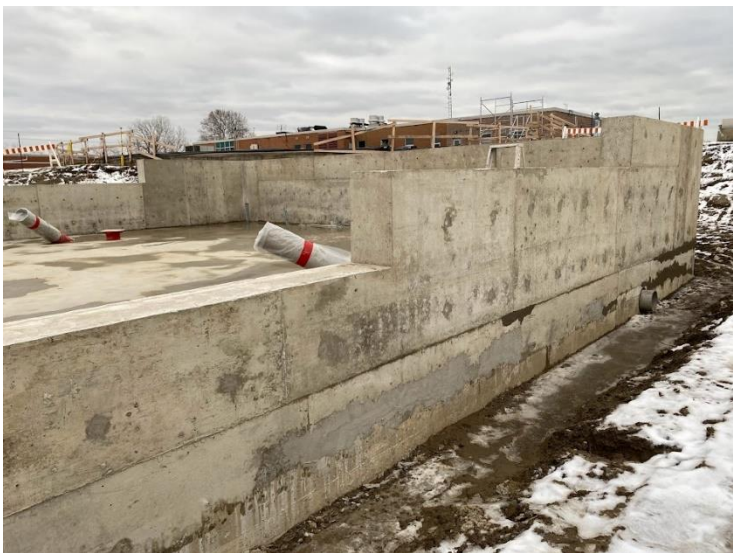
13. Auxiliary Building – Wall Pre Waterproofing & Masonry Repairs in Progress (2022-01-05)
