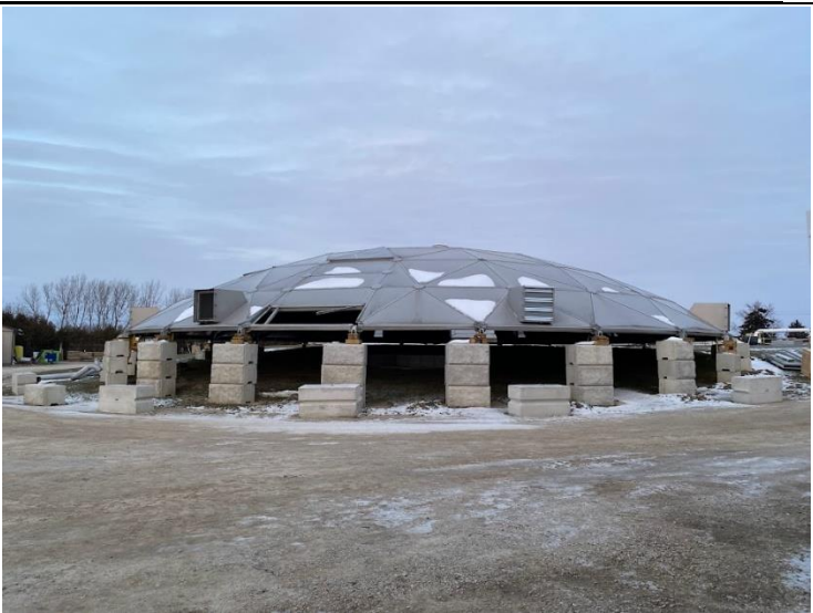
40. Clarifier No. 2 Dome Laydown (2022-01-06)
