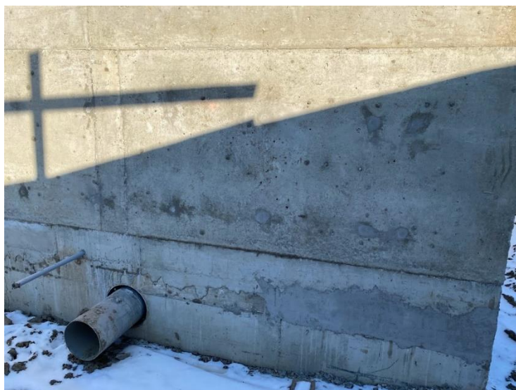
1. Auxiliary Building – Wall Pre Waterproofing & Masonry Repairs in Progress (2022-01-04)
