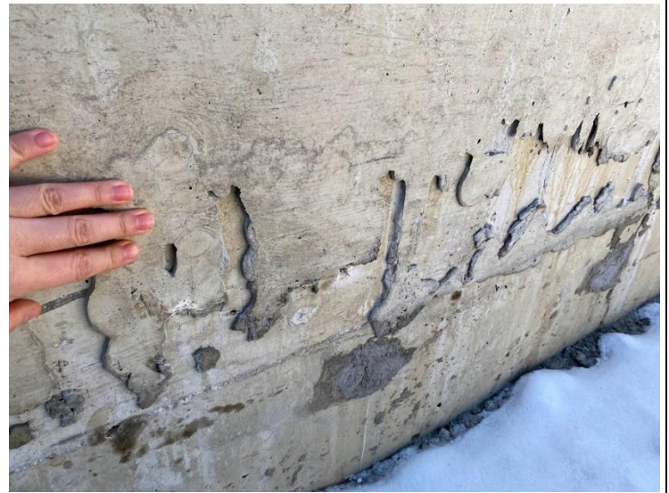
8. Auxiliary Building – Wall Pre Waterproofing & Masonry Repairs in Progress (2022-01-04)
