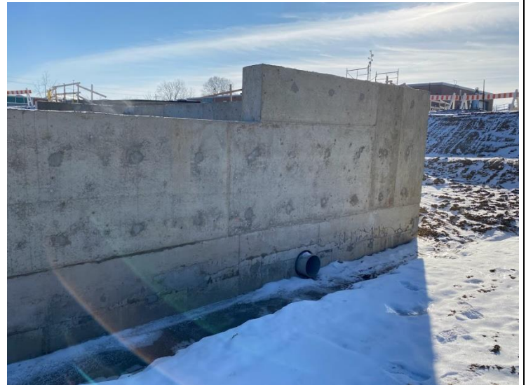
10. Auxiliary Building – Wall Pre Waterproofing & Masonry Repairs in Progress (2022-01-04)
