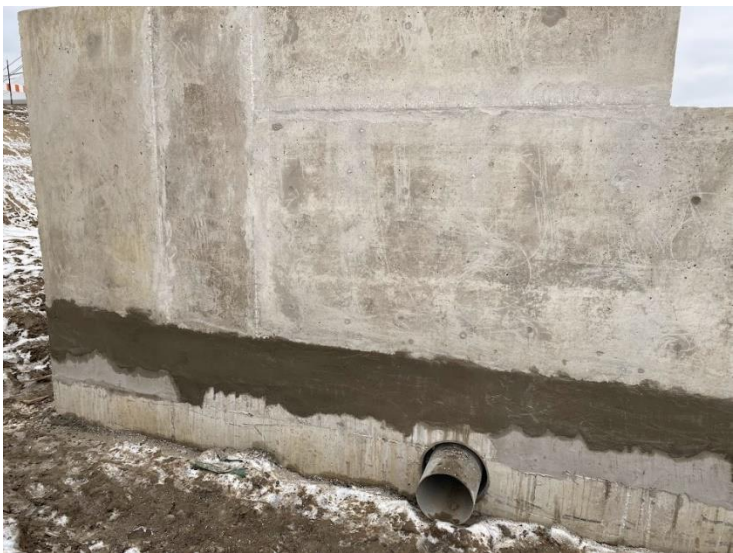
18. Auxiliary Building – Wall Pre Waterproofing & Masonry Repairs in Progress (2022-01-05)
