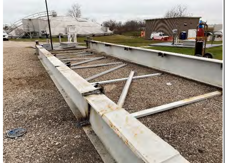
50. Demolition of Clarifier No. 2 Walkway / Beams (2021-12-03)
