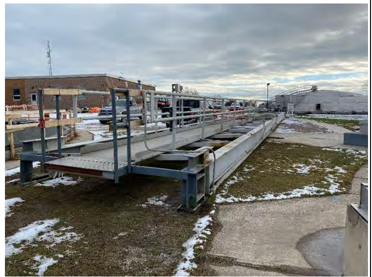
2. Clarifier No. 2 – Removed Walkway (2021-11-29)
