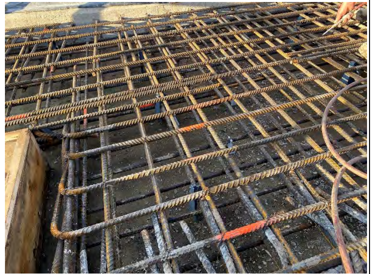
36. Clarifier No. 2 Blowdown Chamber – Rebar for Top Suspended Slab (Pre Compressed Air Cleanout) (2021-12-02)
