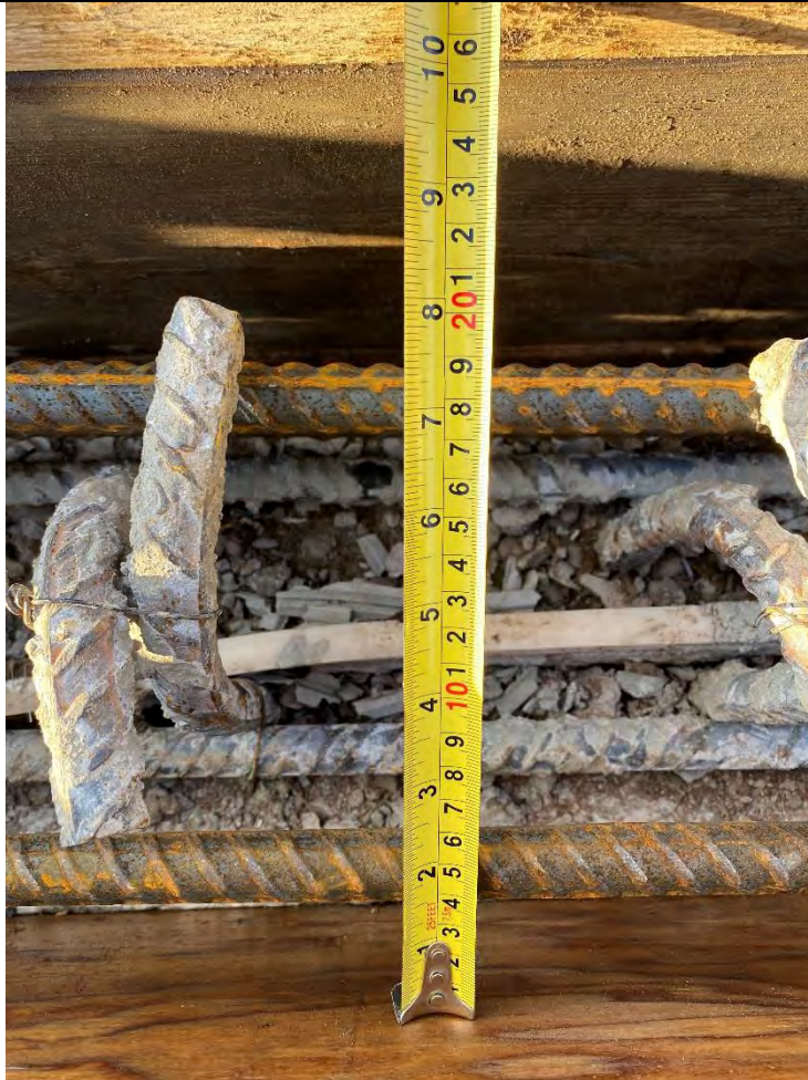
31. Clarifier No. 2 Blowdown Chamber – Rebar for Top Suspended Slab (Pre Compressed Air Cleanout) (2021-12-02)
