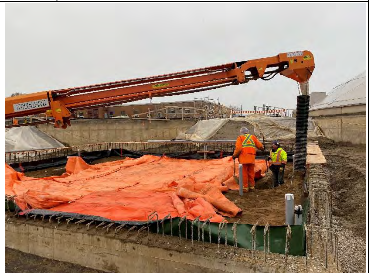
42. Concrete Pour for Auxiliary Building: Mud Mat for Recirculation Piping (2021-12-03)
