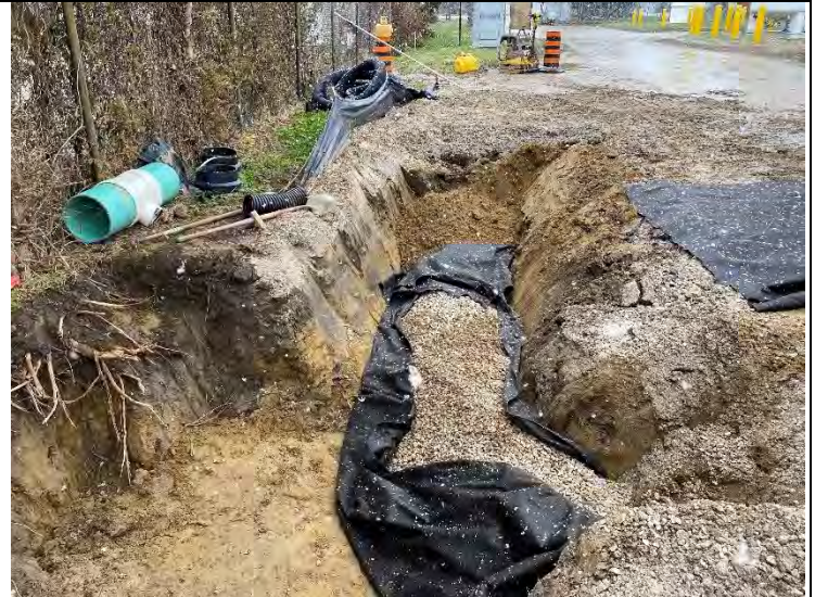
44. Auxiliary Building Foundation Drain – 300 mm Perforated Corrugated Pipe with Clearstone Surrounding on Geotextile (2021-12-03)
