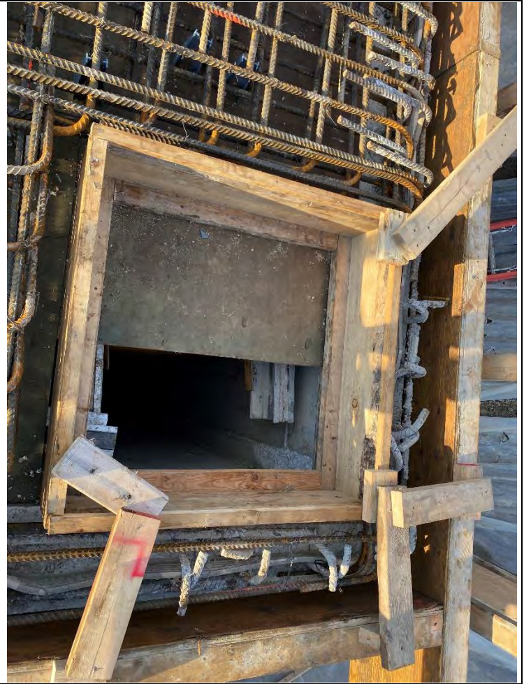
40. Clarifier No. 2 Blowdown Chamber – Equipment Access Hatch (2021-12-02)
