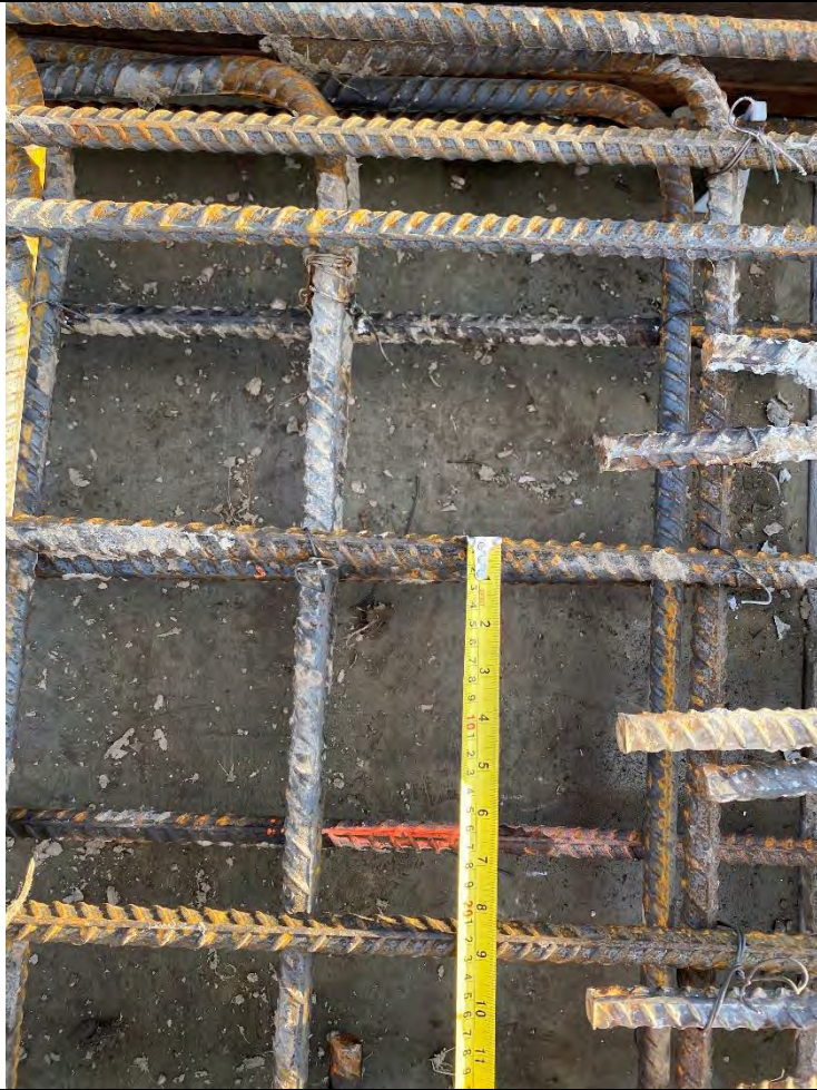
39. Clarifier No. 2 Blowdown Chamber – Rebar for Top Suspended Slab (Pre Compressed Air Cleanout) (2021-12-02)
