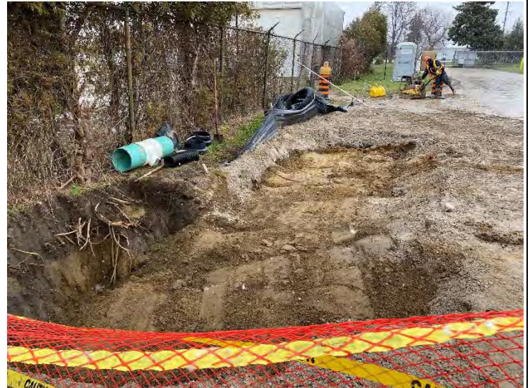
46. Auxiliary Building Foundation Drain – Covered with Earth Fill (2021-12-03)
