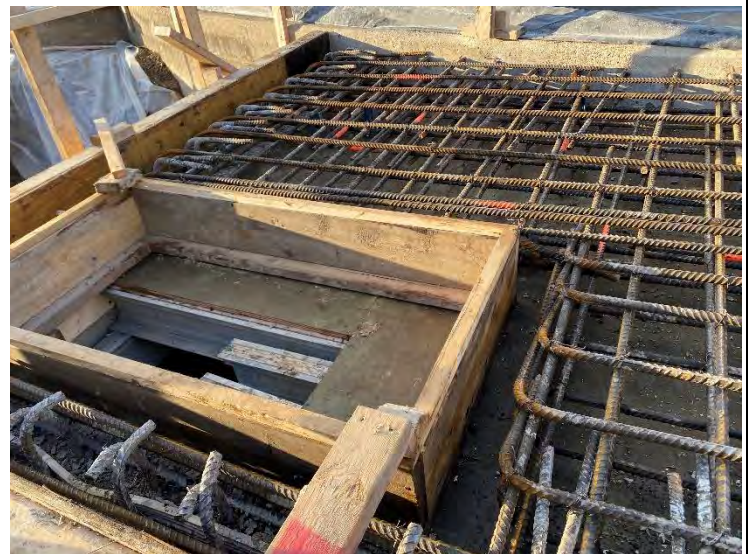
34. Clarifier No. 2 Blowdown Chamber – Rebar for Top Suspended Slab and Access (Pre Compressed Air Cleanout) (2021-12-02)
