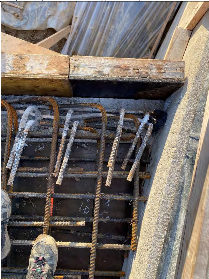
37. Clarifier No. 2 Blowdown Chamber – Rebar for Top Suspended Slab (Pre Compressed Air Cleanout) (2021-12-02)
