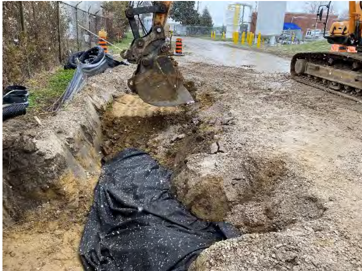
45. Auxiliary Building Foundation Drain – 300 mm Perforated Corrugated Pipe with Clearstone Surrounding on Geotextile (2021-12-03)
