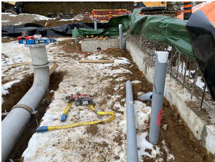
5. Auxiliary Building – Saturation Piping for DAF No. 1 and Plumbing (2021-11-29)
