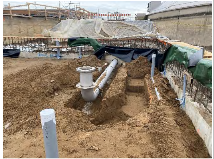
20. Auxiliary Building – Trenching for Recirculation Piping (2021-12-01)
