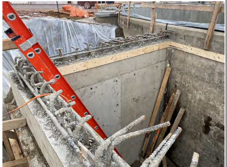
14. Clarifier No. 2 Blowdown Chamber Stripped Forms – Interior (2021-11-30)
