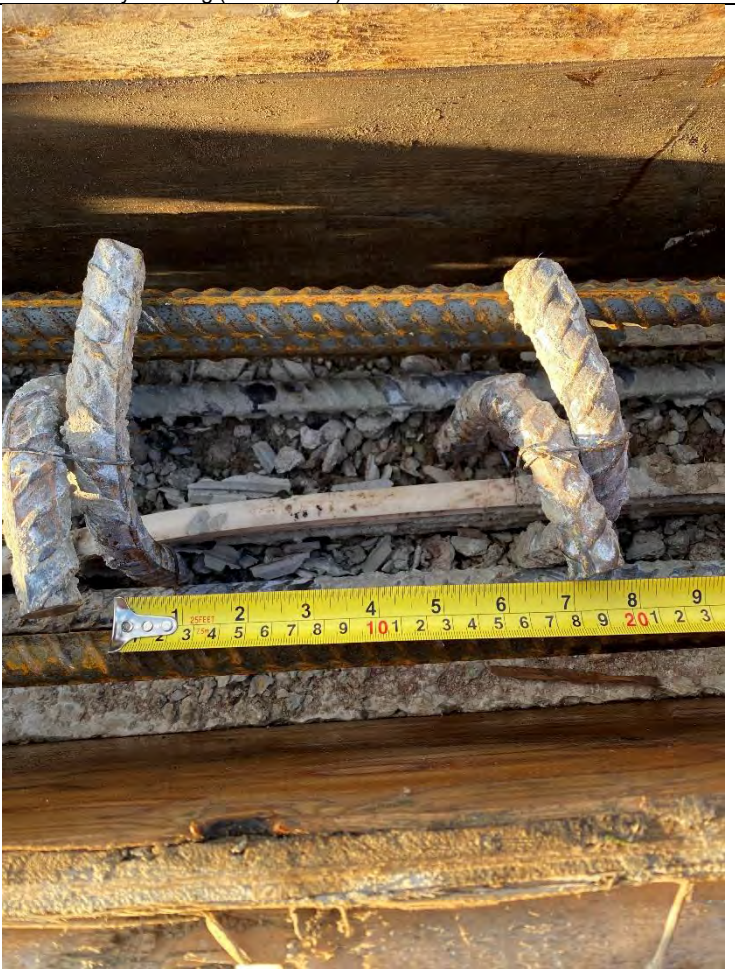
30. Clarifier No. 2 Blowdown Chamber – Rebar for Top Suspended Slab (Pre Compressed Air Cleanout) (2021-12-02)
