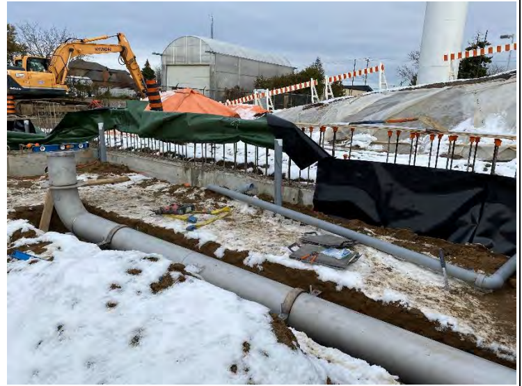
4. Auxiliary Building – Saturation Piping for DAF No. 1 (2021-11-29)
