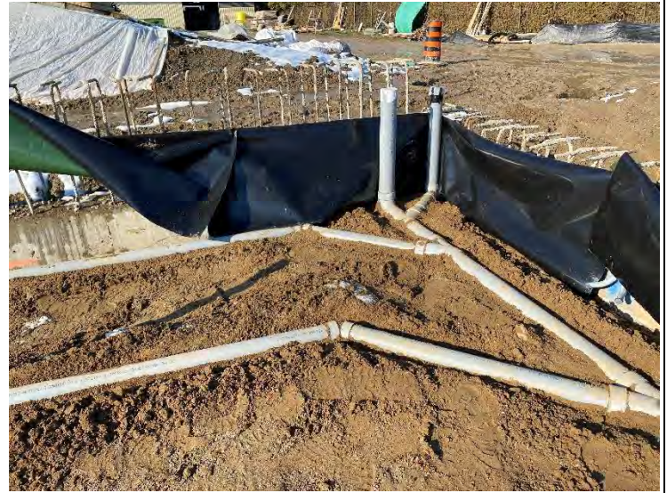
8. Auxiliary Building – Plumbing in Northwest Corner (2021-11-30)
