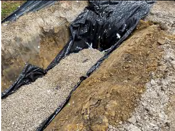
43. Auxiliary Building Foundation Drain – 300 mm Perforated Corrugated Pipe with Clearstone Surrounding on Geotextile (2021-12-03)
