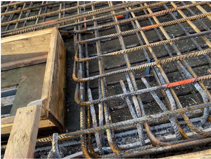
35. Clarifier No. 2 Blowdown Chamber – Rebar for Top Suspended Slab (Pre Compressed Air Cleanout) (2021-12-02)
