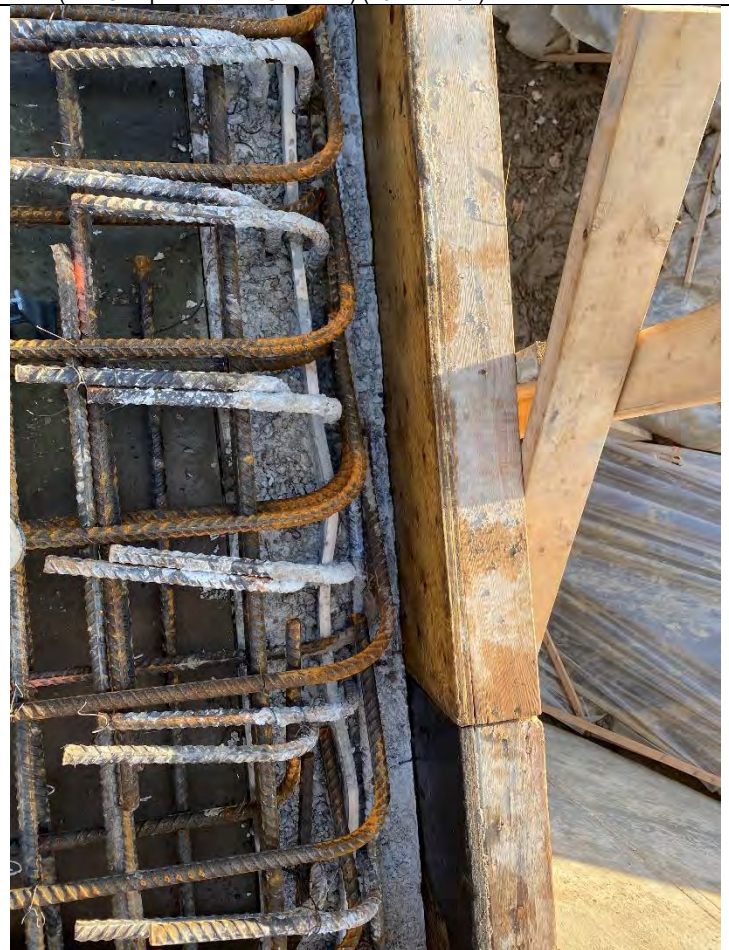
38. Clarifier No. 2 Blowdown Chamber – Rebar for Top Suspended Slab (Pre Compressed Air Cleanout) (2021-12-02)
