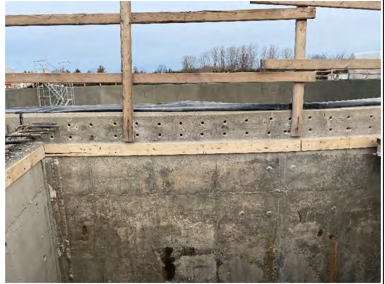
16. Clarifier No. 2 Blowdown Chamber Drilled Holes for Dowels (2021-12-01)
