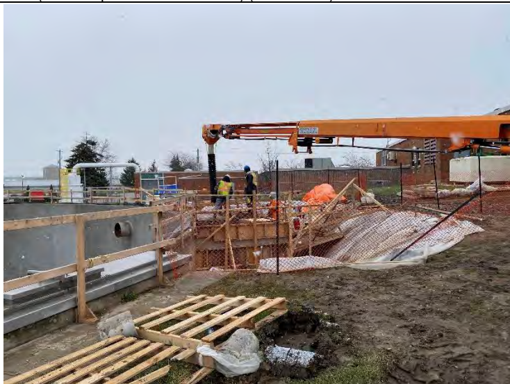
41. Concrete Pour for Clarifier No. 2 Blowdown Chamber – Top Suspended Slab (2021-12-03)
