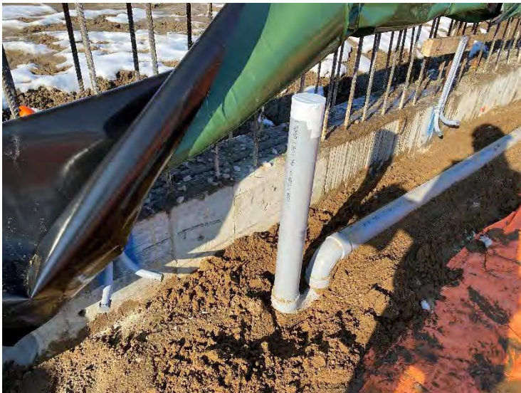
9. Auxiliary Building – Plumbing: P Trap (2021-11-30)
