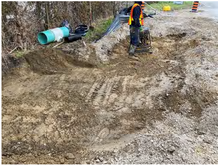
47. Auxiliary Building Foundation Drain – Covered with Earth Fill and Compacted (2021-12-03)
