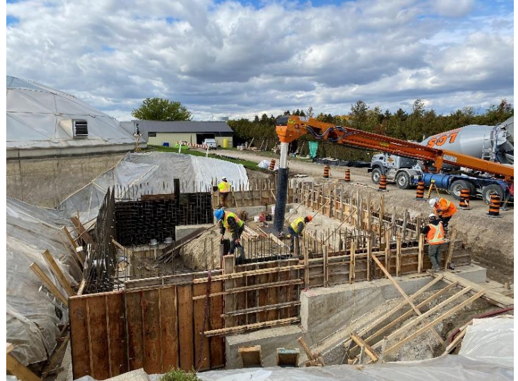
24. Auxiliary Building – Concrete Pour for East and West Step Foundations and North Wall Below Grade (2021-11-01)
