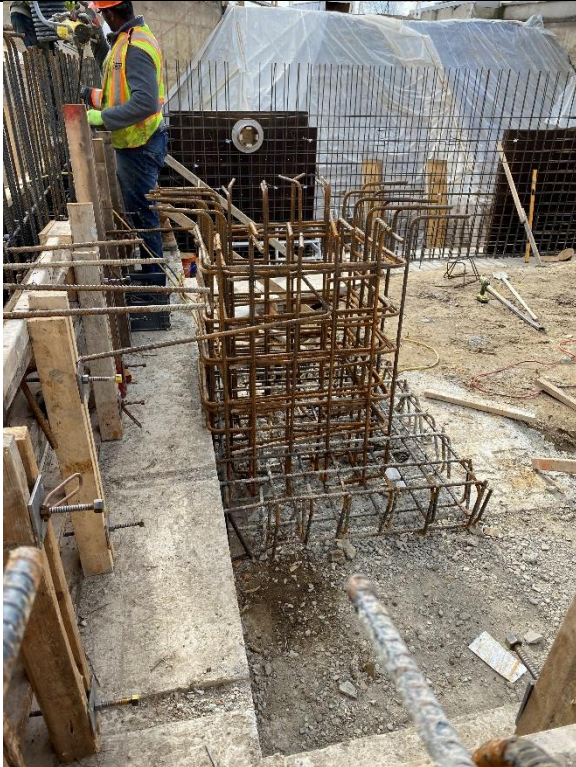
25. Auxiliary Building – Sump Pit Rebar (2021-11-01)
