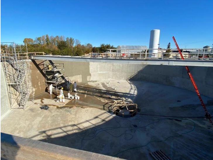
35. Clarifier No. 2 – Gem Plast TC for Interior Wall Coating in Progress (2021-11-03)
