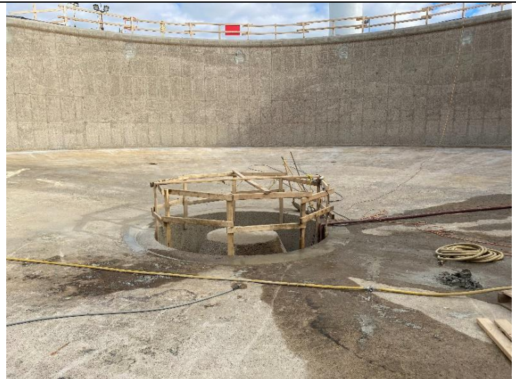
10. Clarifier No. 2 – Sludge Blowdown Cone (2021-11-01)
