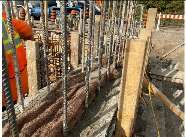
28. Auxiliary Building – Concrete Pour: East Step Foundations Below Grade (2021-11-01)
