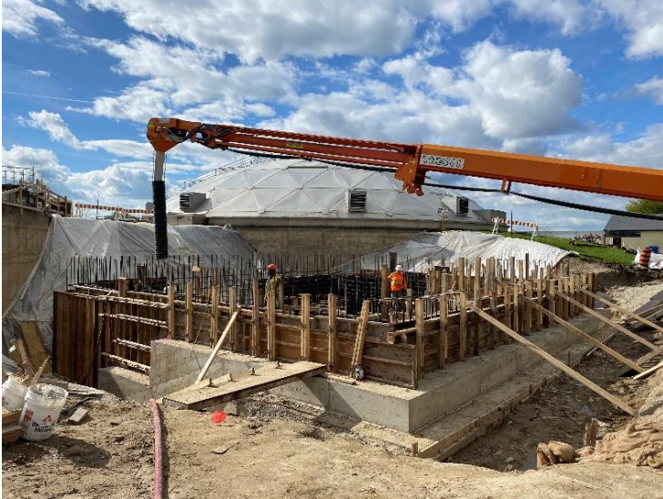
23. Auxiliary Building – Concrete Pour for East and West Step Foundations and North Wall Below Grade (2021-11-01)
