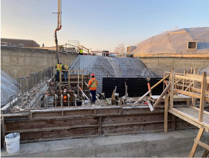
47. Auxiliary Building – Concrete Pour for Below Grade South and Southeast Wall (2021-11-05)
