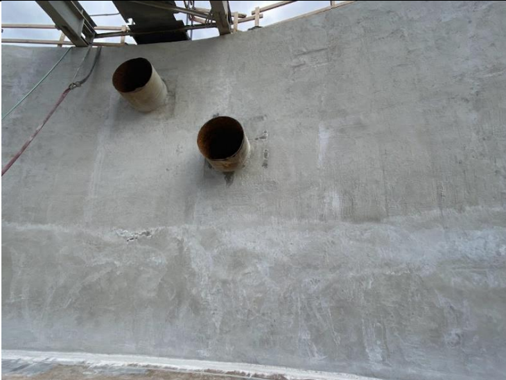
33. Clarifier No. 2 – Gem Plast TC for Interior Wall Coating in Progress (2021-11-02)
