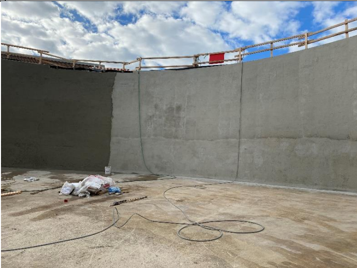
13. Clarifier No. 2 – Gem Plast TC for Interior Wall Coating in Progress (2021-11-01)
