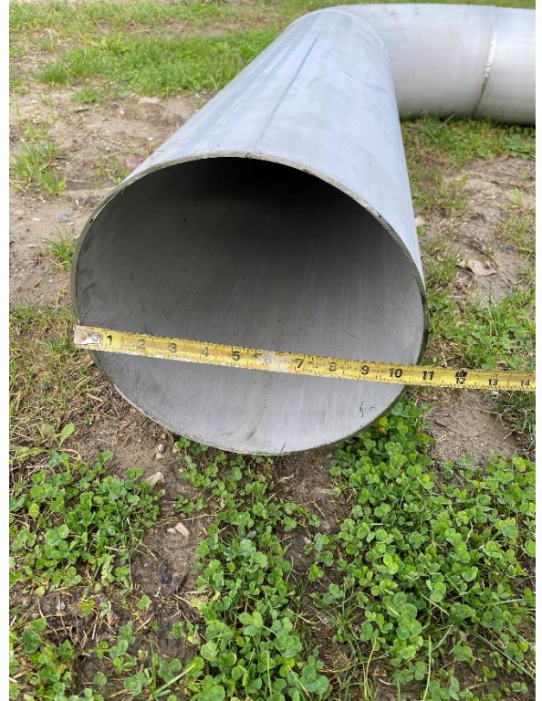
20. Process Piping – 316 SS for the Saturation and Recycle Line Delivered (2021-11-01)
