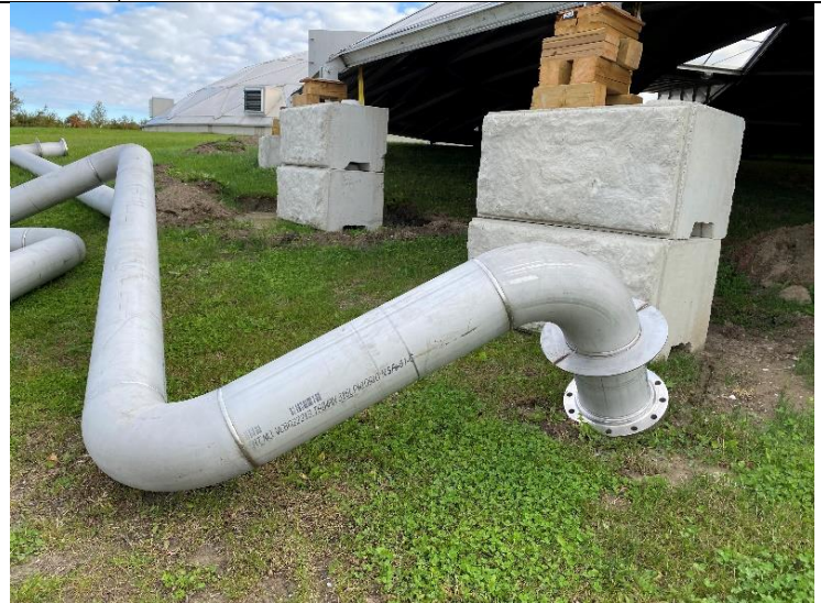
22. Process Piping – 316 SS for the Saturation and Recycle Line Delivered (2021-11-01)
