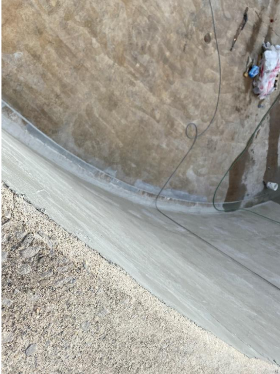
19. Clarifier No. 2 – Gem Plast TC for Interior Wall Coating in Progress up to the Top of the Clarifier Tank (2021-11-01)
