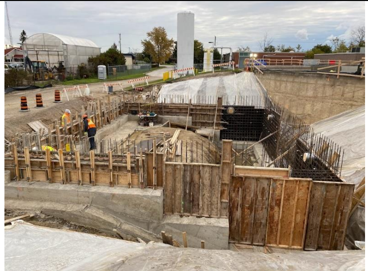
32. Auxiliary Building – Formwork for Below Grade walls in Progress (2021-11-02)
