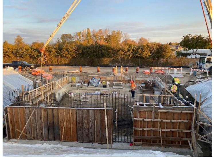
48. Auxiliary Building – Concrete Pour for Below Grade South and Southeast Wall (2021-11-05)
