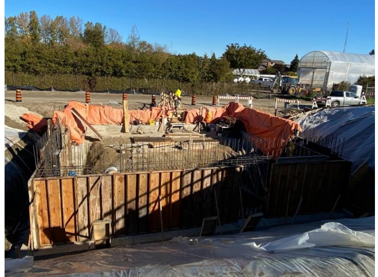
36. Auxiliary Building – Formwork for Below Grade walls in Progress (2021-11-03)
