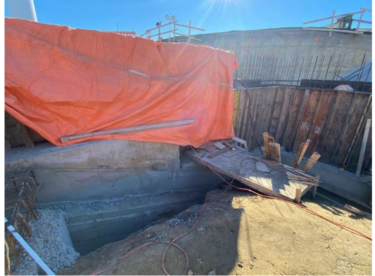
38. Auxiliary Building – Southeast Corner Formwork for Below Grade Walls (2021-11-03)
