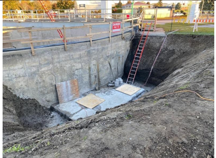
34. Clarifier No. 2 – Blowdown Chamber Cores and Subsequent Saw Cutting Complete (2021-11-02)
