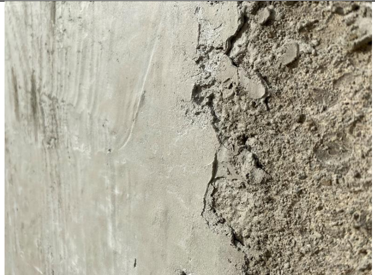
14. Clarifier No. 2 – Transition from Substrate to Gem Plast TC for Interior Wall: Coating in Progress (2021-11-01)
