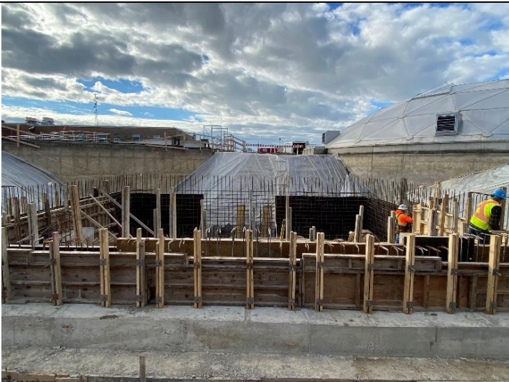
9. Auxiliary Building – Rebar and Formwork Installations (2021-11-01)
