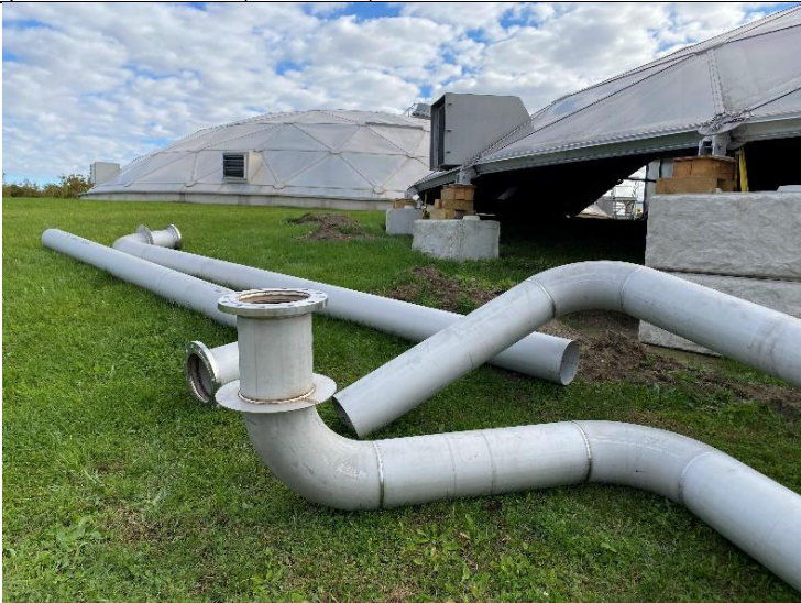
21. Process Piping – 316 SS for the Saturation and Recycle Line Delivered (2021-11-01)
