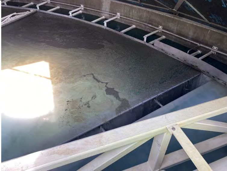
49. DAF No. 1: In Service Mode with Partial Flow to Waste (2022-09-21)
