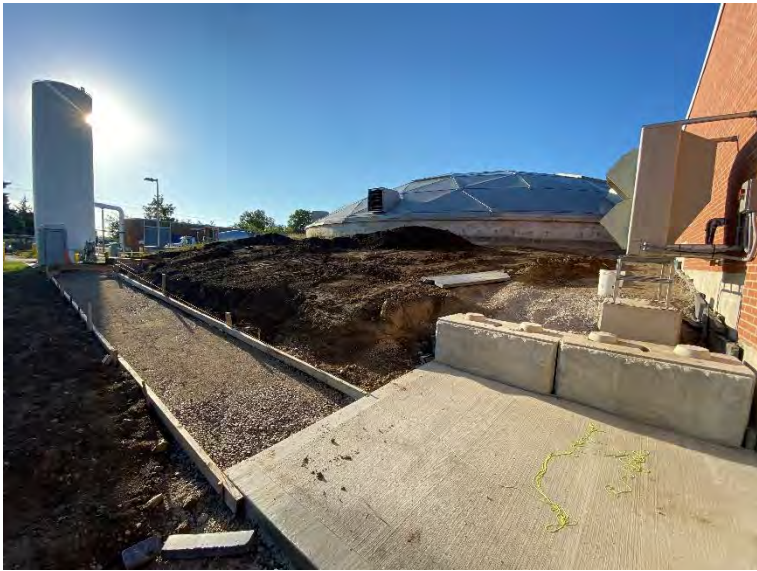
16. Sidewalk and Step Formwork from DAF No. 1 Tank to Auxiliary Equipment Building (2022-09-21)
