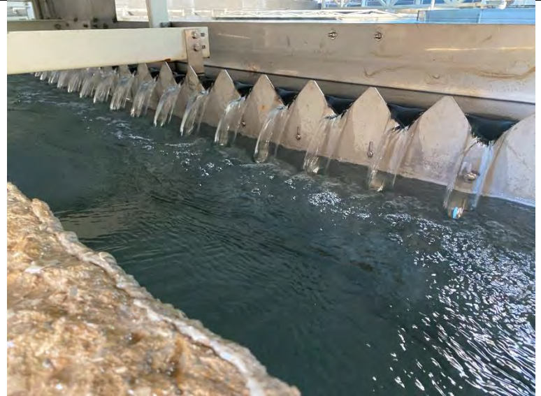
30. DAF No. 1 Effluent Troughs at Overflow (2022-09-21)
