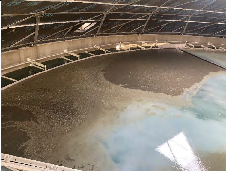
47. DAF No. 1: In Service Mode with Partial Flow to Waste (2022-09-21)
