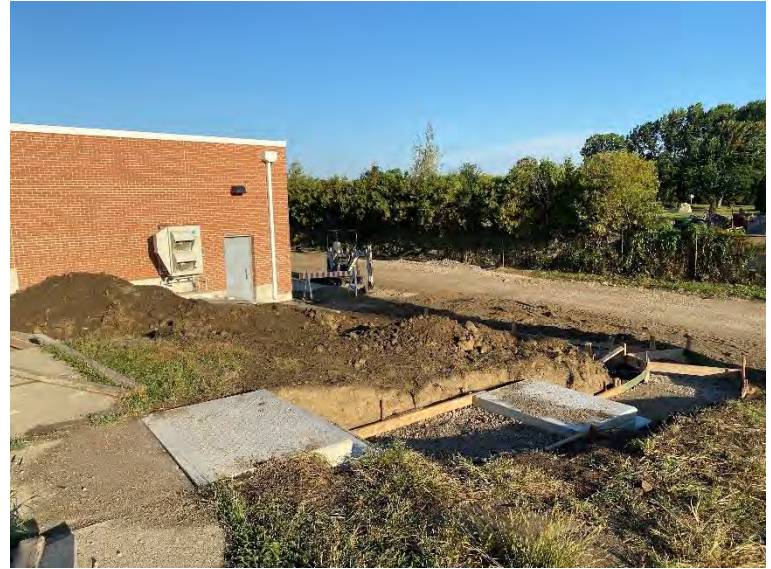
12. Sidewalk and Step Formwork from DAF No. 1 Tank to Auxiliary Equipment Building (2022-09-21)
