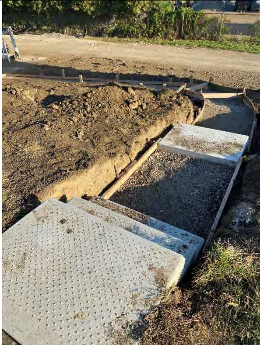
13. Sidewalk and Step Formwork from DAF No. 1 Tank to Auxiliary Equipment Building (2022-09-21)
