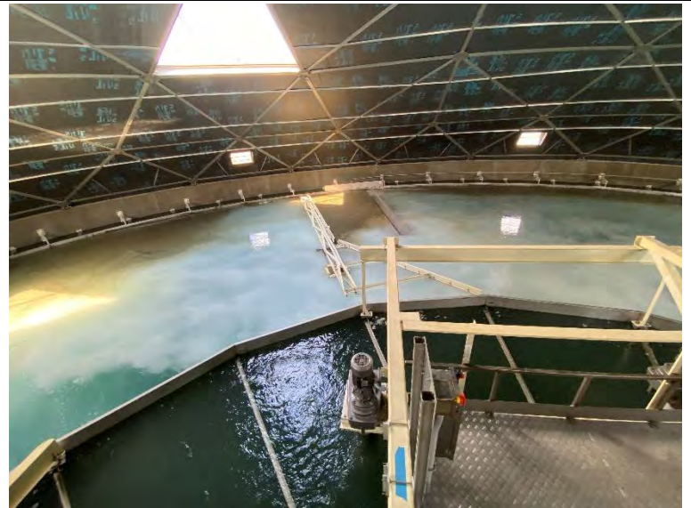
54. DAF No. 1: In Service Mode with Partial Flow to Waste (2022-09-21)
