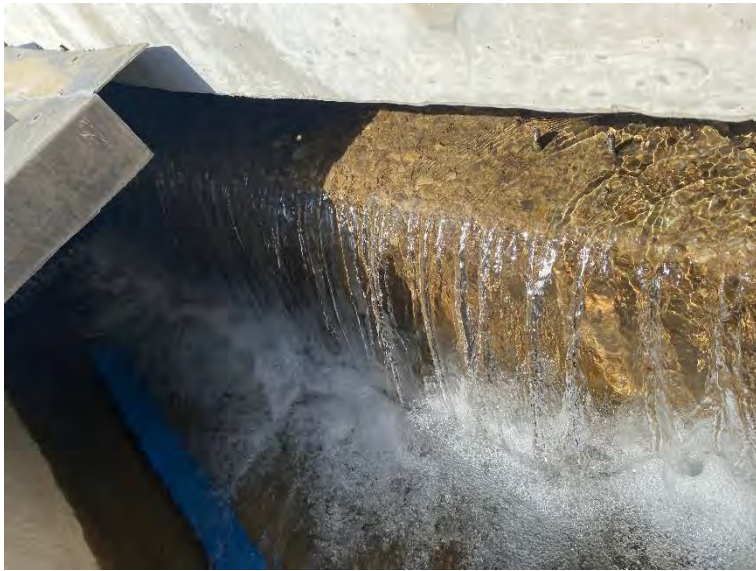
51. DAF No. 1 at Overflow: In Service Mode with Partial Flow to Waste (2022-09-21)
