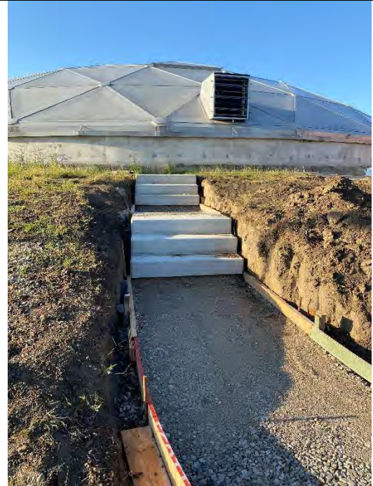
14. Sidewalk and Step Formwork from DAF No. 1 Tank to Auxiliary Equipment Building (2022-09-21)
