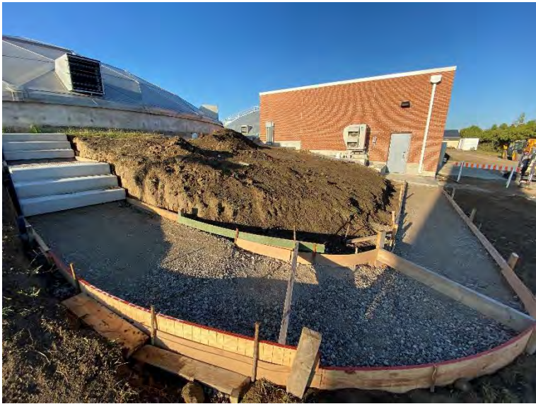
15. Sidewalk and Step Formwork from DAF No. 1 Tank to Auxiliary Equipment Building (2022-09-21)
