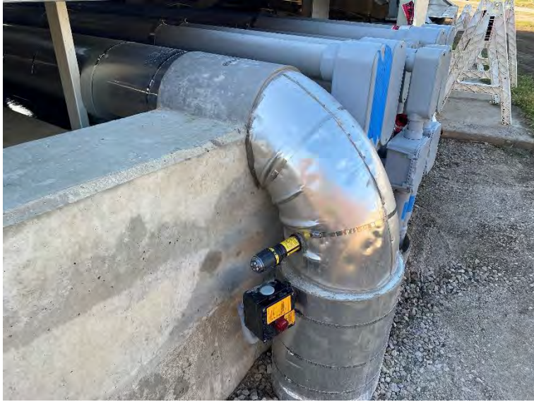
23. Saturation Piping from Auxiliary Equipment Building to DAF No. 1 Tank (2022-09-21)
