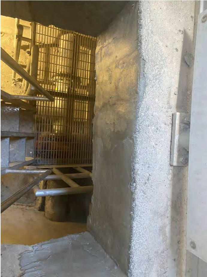
85. DAF No. 1 Blowdown Chamber: Concrete Repair on Opening Through Slab from 1 st Level to 2 nd Level (2022-09-23)
