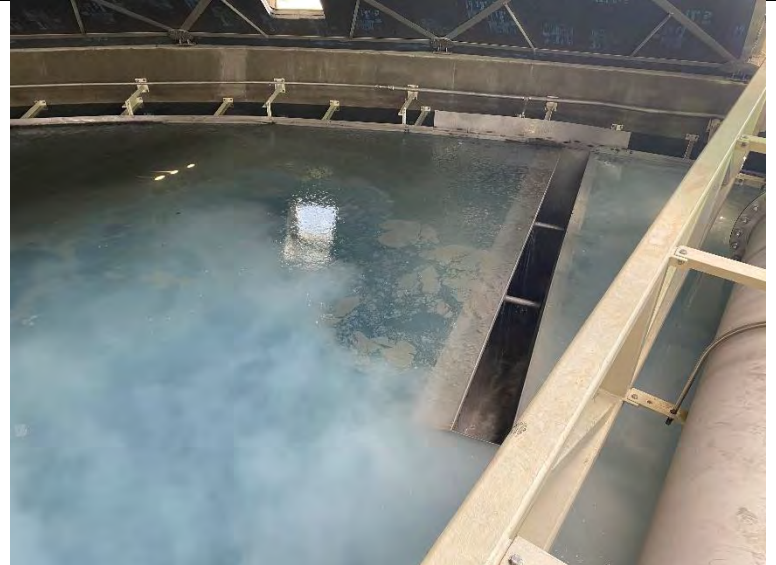
66. DAF No. 1: In Service Mode with Partial Flow to Waste (2022-09-22)
