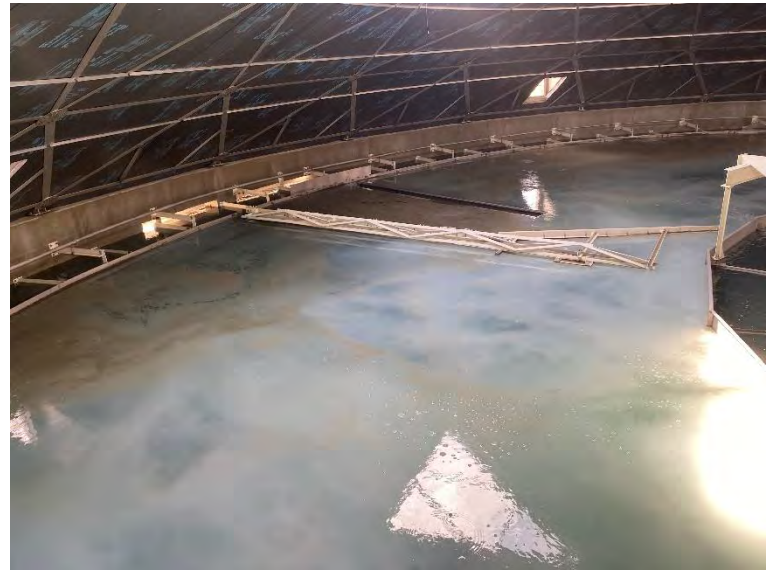
52. DAF No. 1: In Service Mode with Partial Flow to Waste (2022-09-21)
