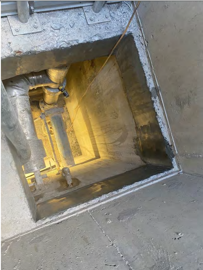
80. DAF No. 1 Blowdown Chamber: Concrete Repair on Opening Through Slab from 1 st Level to 2 nd Level (2022-09-23)
