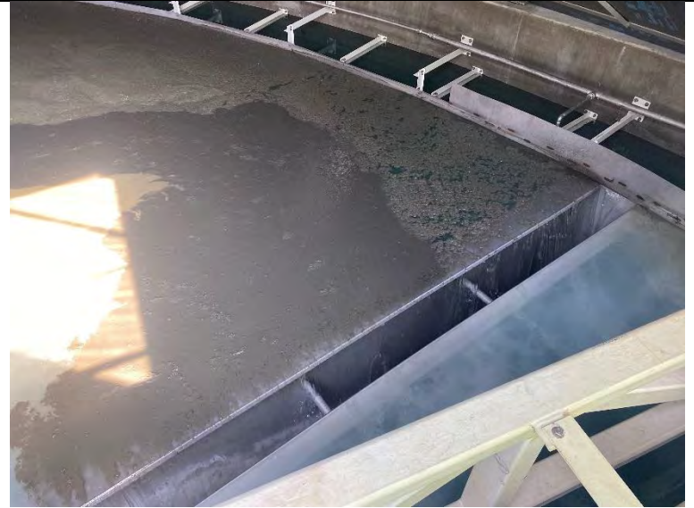
48. DAF No. 1: In Service Mode with Partial Flow to Waste (2022-09-21)
