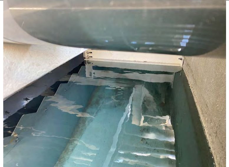
50. DAF No. 1: In Service Mode with Partial Flow to Waste (2022-09-21)
