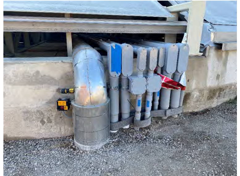
22. Saturation Piping from Auxiliary Equipment Building to DAF No. 1 Tank (2022-09-21)
