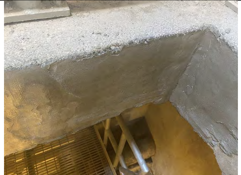
84. DAF No. 1 Blowdown Chamber: Concrete Repair on Opening Through Slab from 1 st Level to 2 nd Level (2022-09-23)
