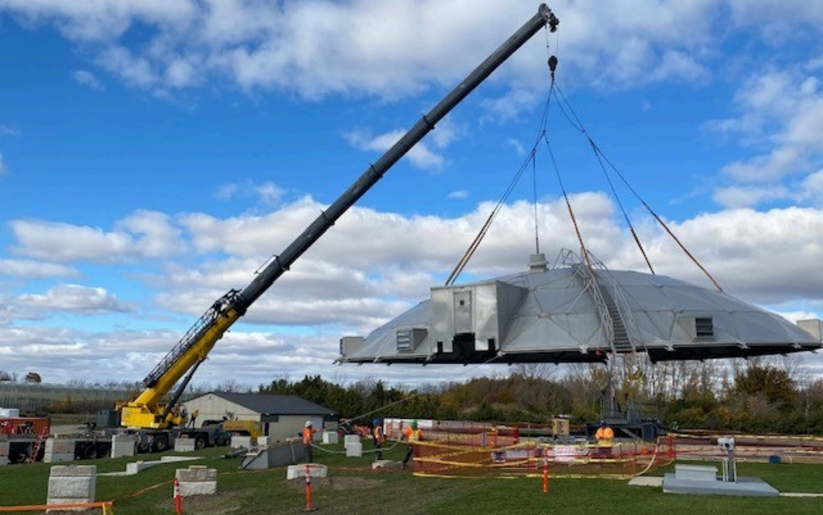
DAF #2 UNIT INSTALLATION, FALL 2024 RUTHVEN WATER TREATMENT PLANT
