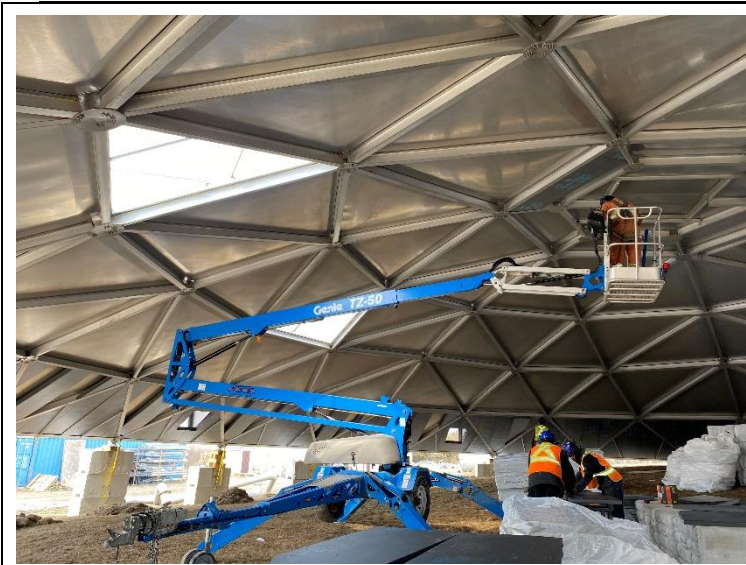
29. Dome Interior Insulation Installation (2022-03-03)
