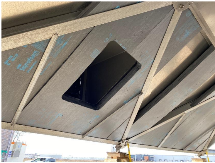
32. Dome Interior Insulation Installation (2022-03-03)
