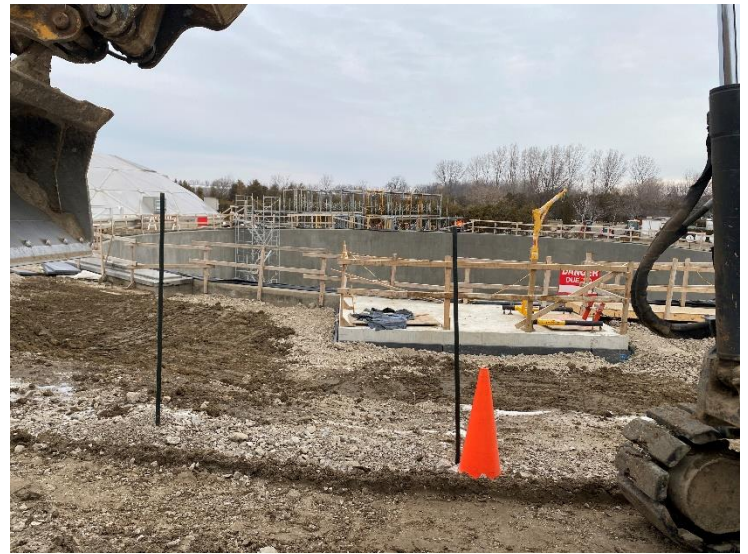
10. Blowdown Chamber Backfill (2022-03-01)
