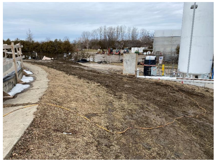
4. Trenching Backfill – WTP to Pull Box to Auxiliary Building (2022-02-28)
