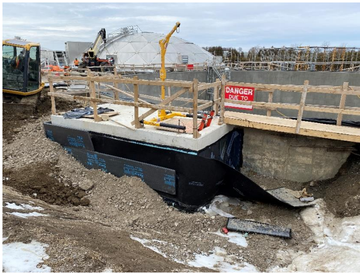
1. Blowdown Chamber – Insulation and Backfill (2022-02-28)
